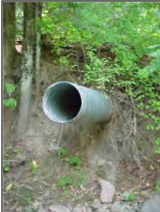
Figure 12 Hanging culvert on back-channel
