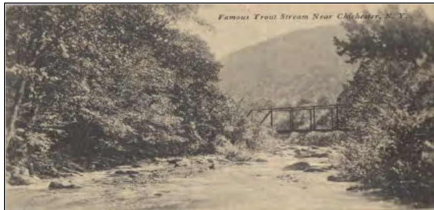
Figure 2 Looking upstream under the NYS Route 214 bridge at Chichester, Courtesy of the Gale Collection
