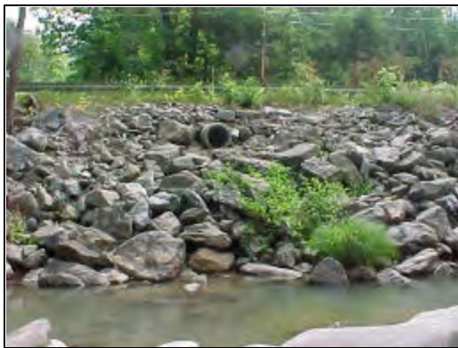
Figure 15 Rip-Rap and Culvert
