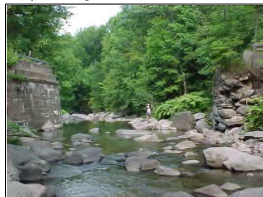
Figure 11 Abandoned Railroad Abutments
