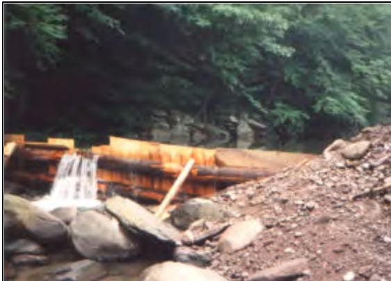
Figure 3 Temporary Pool Digger
