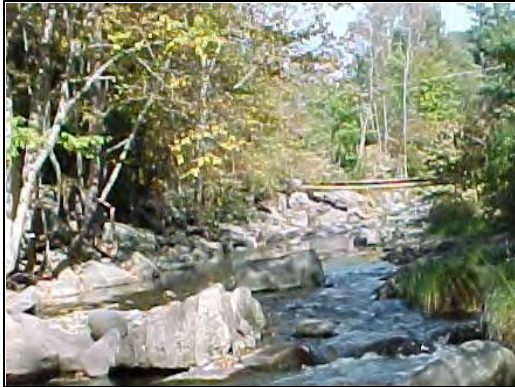
Figure 6 Rip-rap on right bank looking upstream
