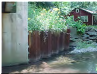
Figure 11 Sheet Piling
