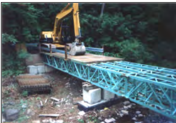
Figure 4 Bridge at Stony Clove Lane under construction, September 16, 1993
