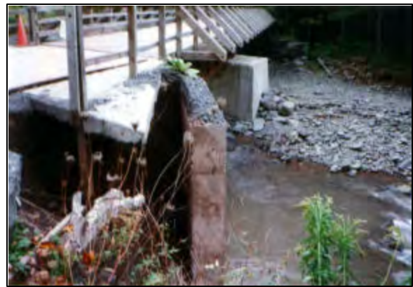
Figure 5 1999 Grubman Road Bridge damage to abutment
