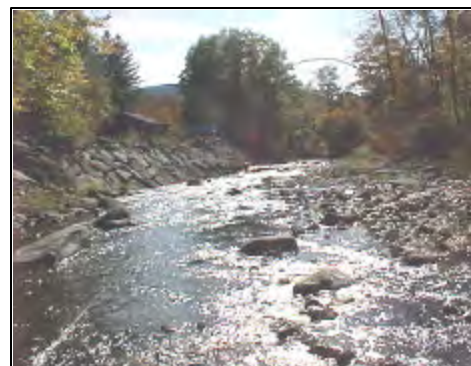
Figure 10 Rip-rap left bank
