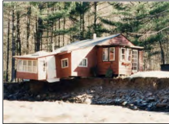
Figure 4 House undermined by bank erosion during the January 1996 flood
