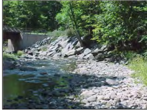
Figure 13 Rip-rap upstream from bridge
