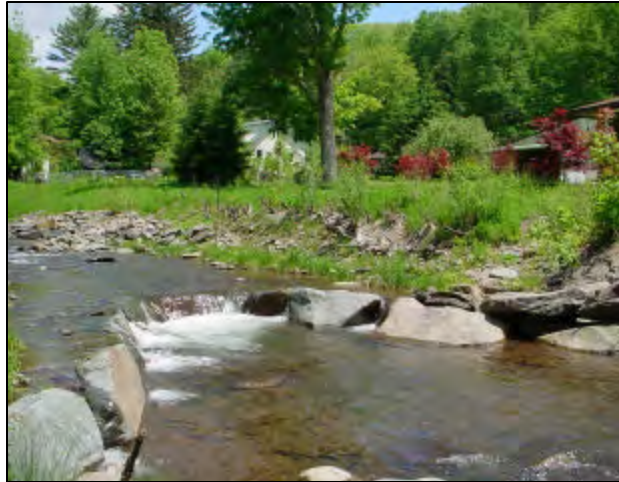
Figure 19 A cross vane at the stream restoration site on Broadstreet Hollow. Notice how the cross vane redirects stream flow into the center of the channel, away from the banks.
