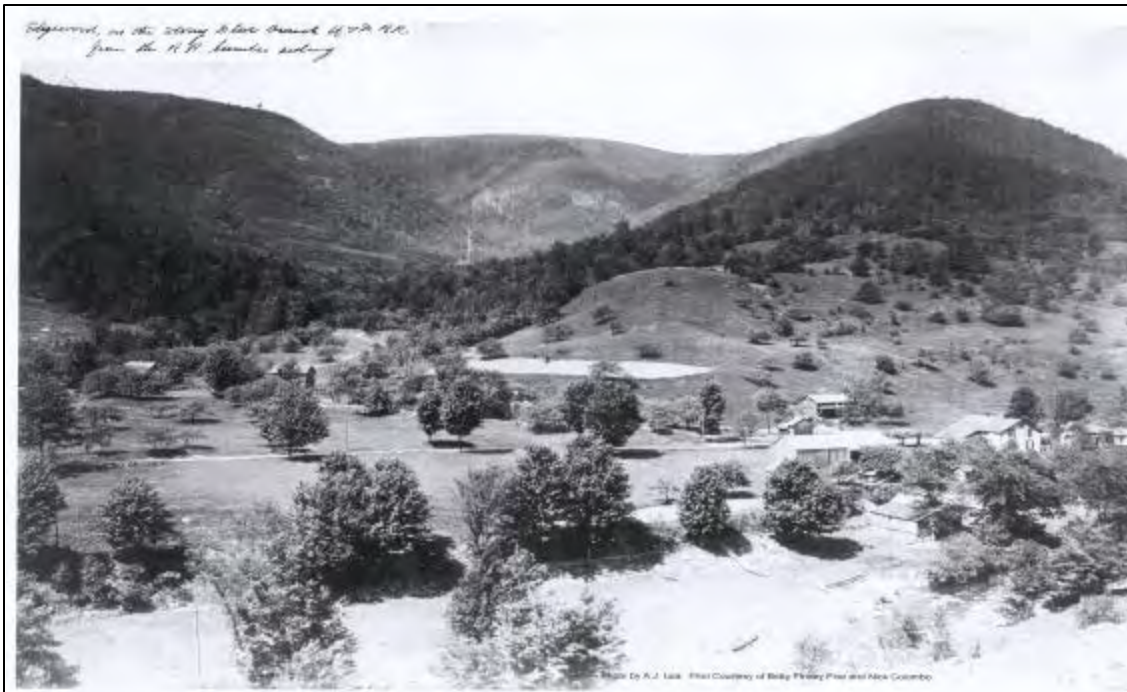
Figure 3 View from railroad line, across Stony Clove Creek and NYS Route 214 in the vicinity of Management Unit 5 - Courtesy of the Gale Collection
