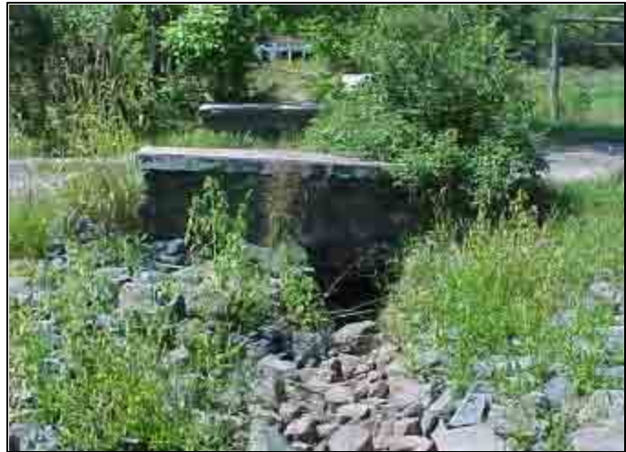
Blocked and buried inlet of upstream culvert.
