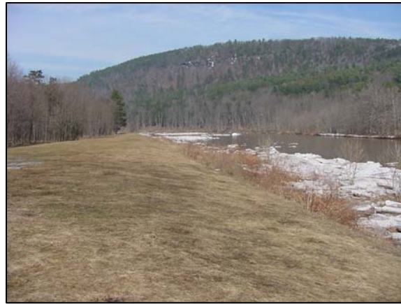
Prattsville flood remediation project pre-construction
