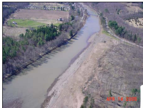
Prattsville flood remediation project post-flood
