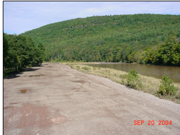
Prattsville flood remediation project post construction
