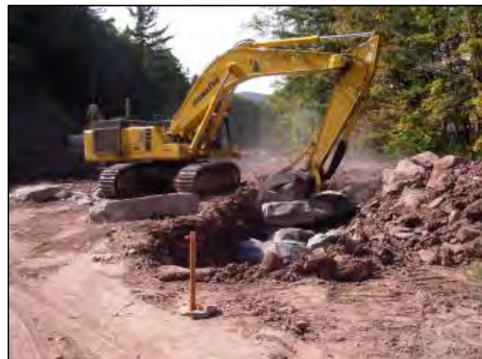
Excavation and construction of a cross vane arm near the center of project reach.
