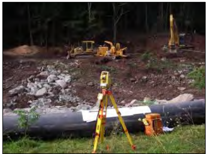
Clearing and grubbing of Phase II.
