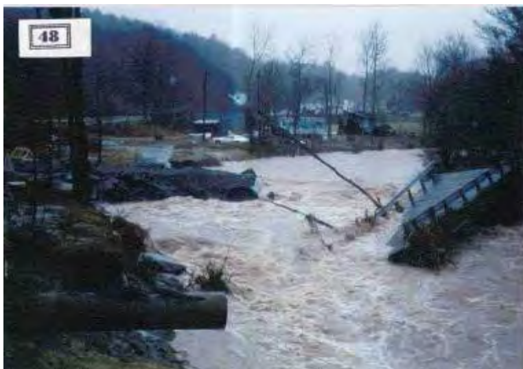
Long Road Bridge during a 1996 flood event.
