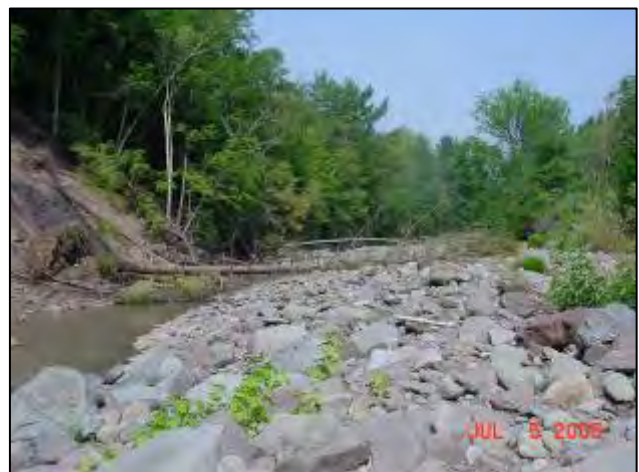
View looking downstream at bank failure and cobble bar.
