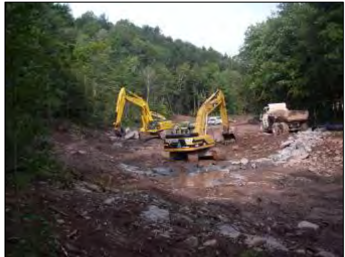
Phase I stream channel excavation.
