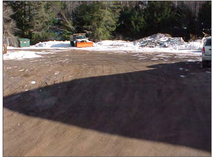
Figure 1. Existing parking area condition.
