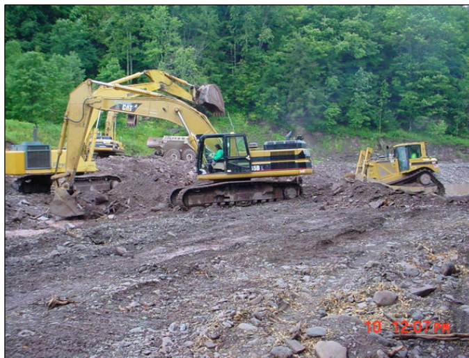
Phase I stream channel excavation.
