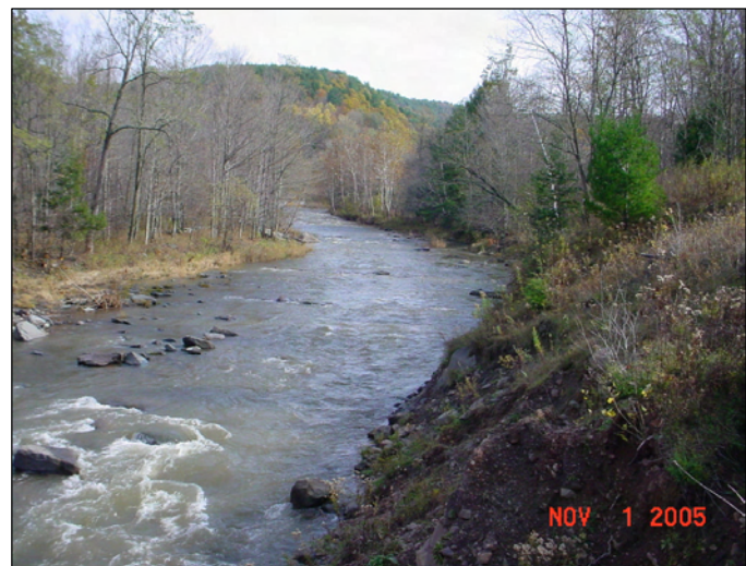
Upstream reach displaying general stability.
