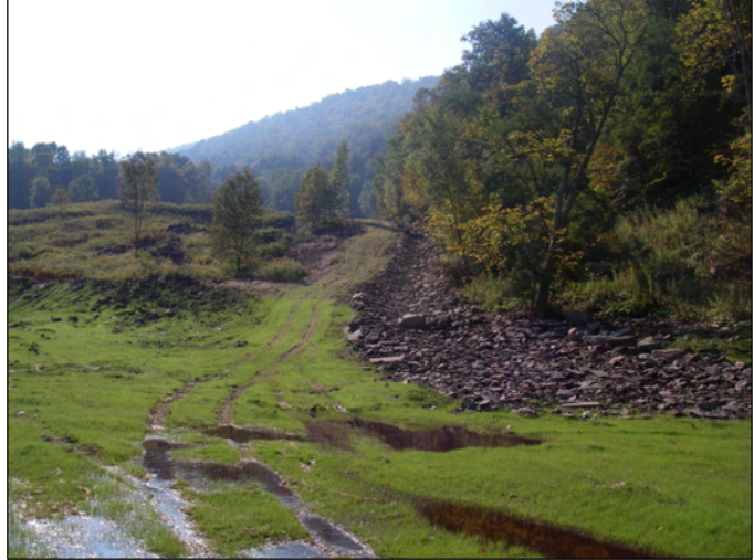
Stabilized borrow area access road and channel.
