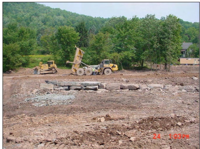
Completed arm of the downstream cross vane.
