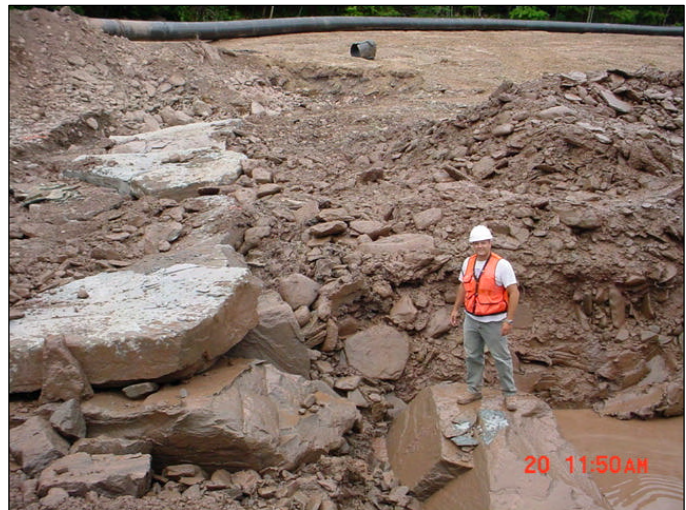
Excavation and construction of a cross vane sill near the center of project reach.
