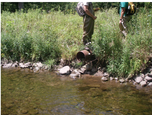
Piped outfall conveying drainage through unstabilized bank (IMGP0352)
