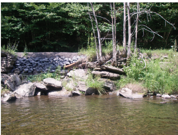
Sloped stone revetment (IMPG344)
