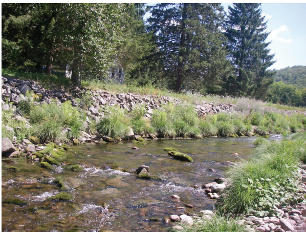
Dumped rip rap revetment (IMPG0331)
