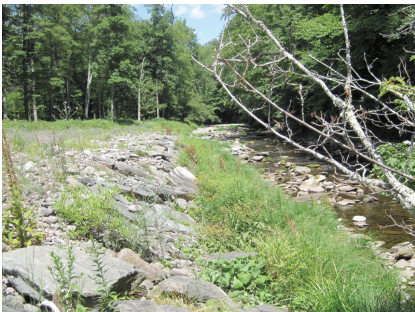
Stacked rock revetment on right bank (A71)
