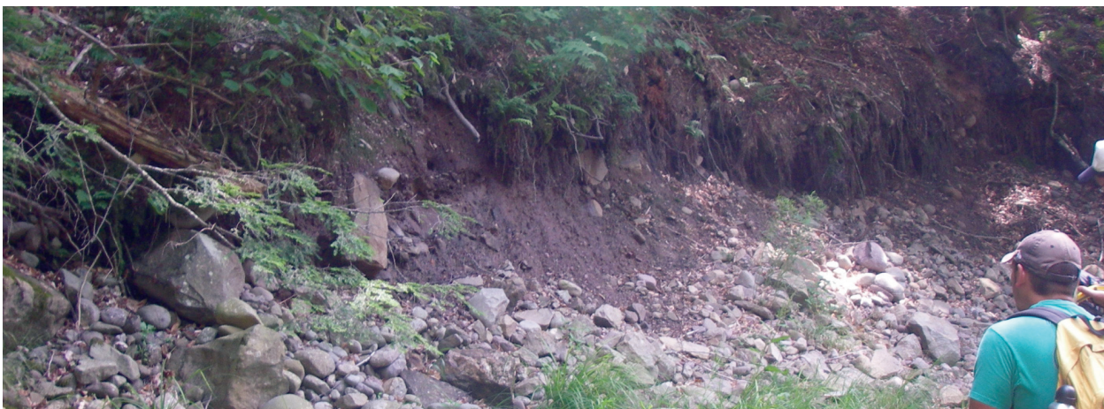
Actively eroding right bank (IMG0368)
