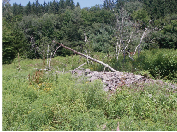
Relict bridge abutment in floodplain (IMG0310)
