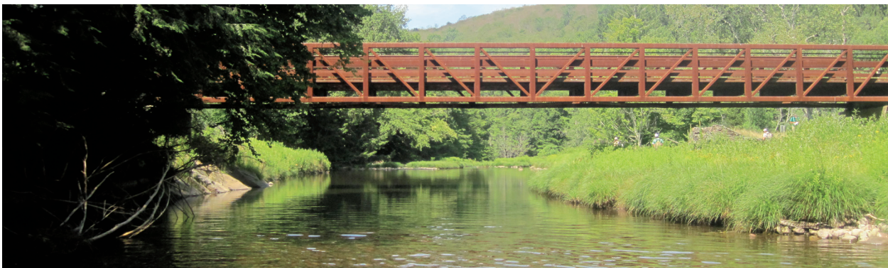
Private bridge on Frost Valley YMCA property (A26)
