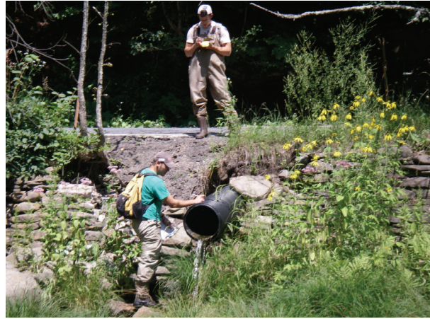
Piped outfall conveying drainage from Frost Valley Road (IMGP0338)
