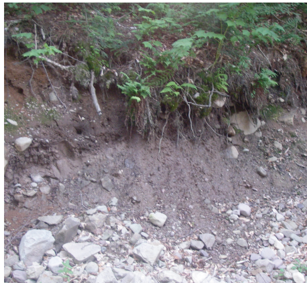
Actively eroding right bank (IMG0369)
