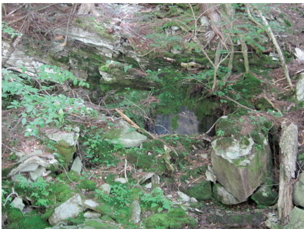
Groundwater seeps from left valley wall (A67)
