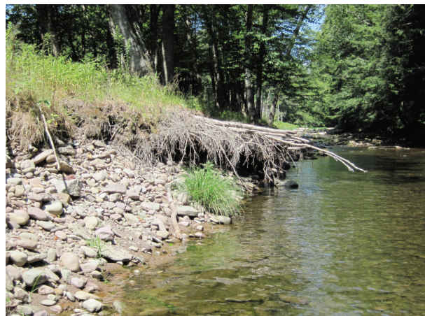
Hydraulic erosion undercutting right bank (A76)
