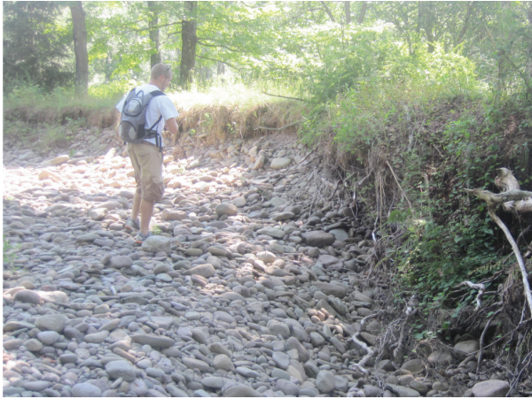
Eroding left bank (A38)
