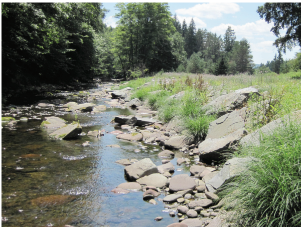
Stacked rock revetment on right bank (A70)
