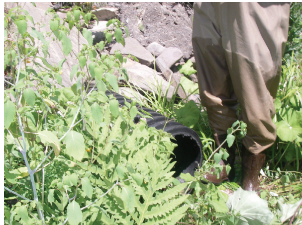
Piped outfall conveying drainage from Frost Valley Road (IMGP0341)
