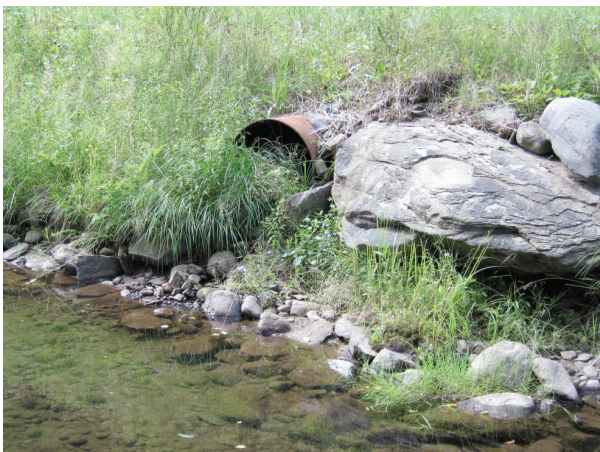
Piped outfall conveying flow into side channel (A85)
