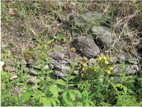
Rip-rap and gabion baskets along right bank (A91)
