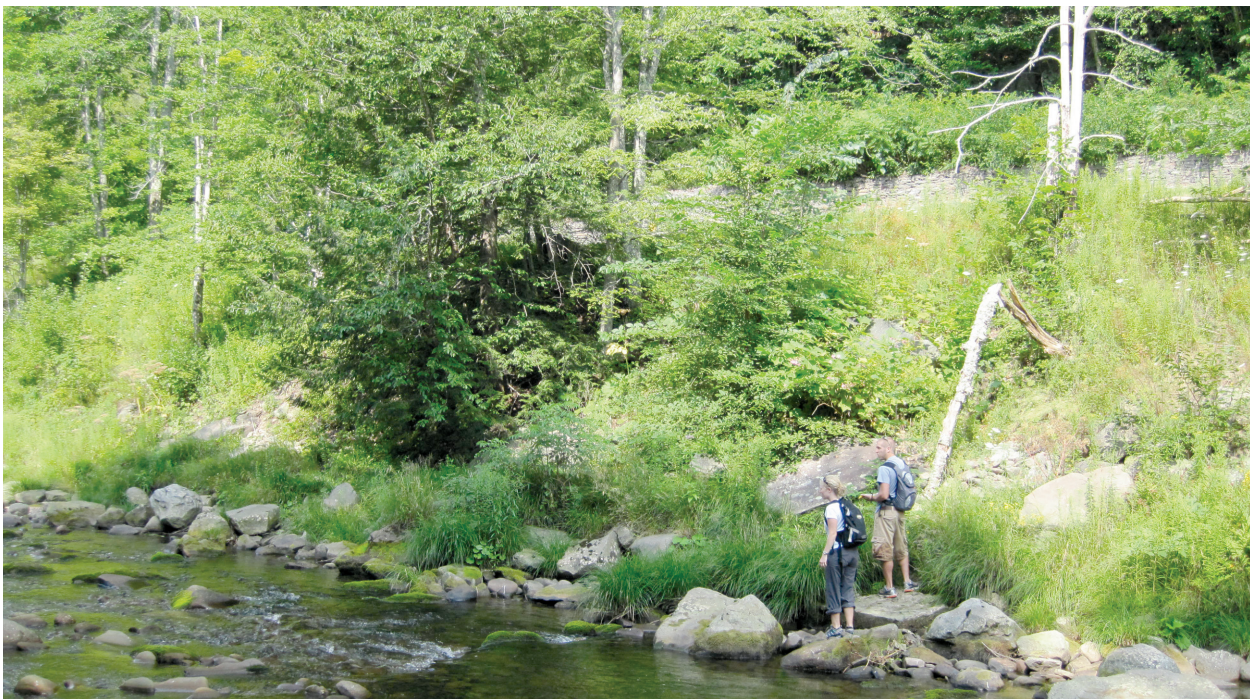
Dumped rock and stacked rock revetment (A99)
