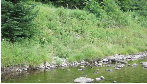
Vegetated stacked rock revetment (A106)
