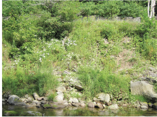
Stacked rock revetment (A101)
