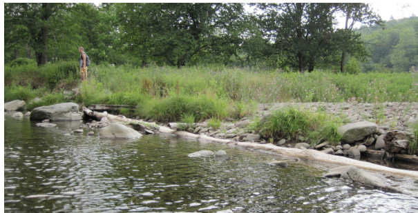
Log cribbing rip-rap (A111)
