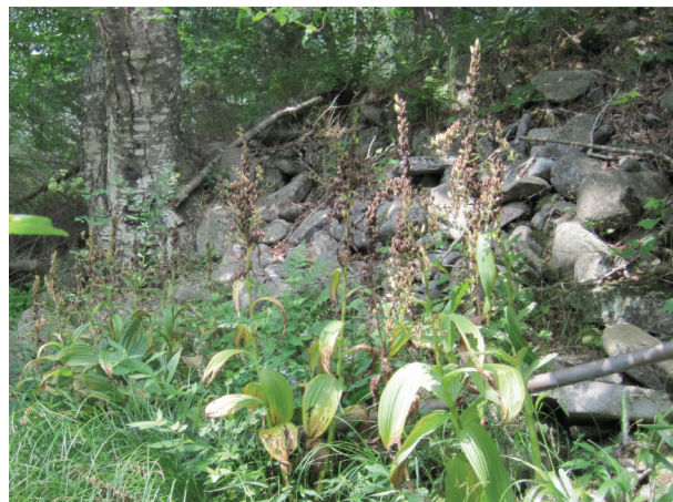
Rip-rap revetment protecting Frost Valley Road (A131)
