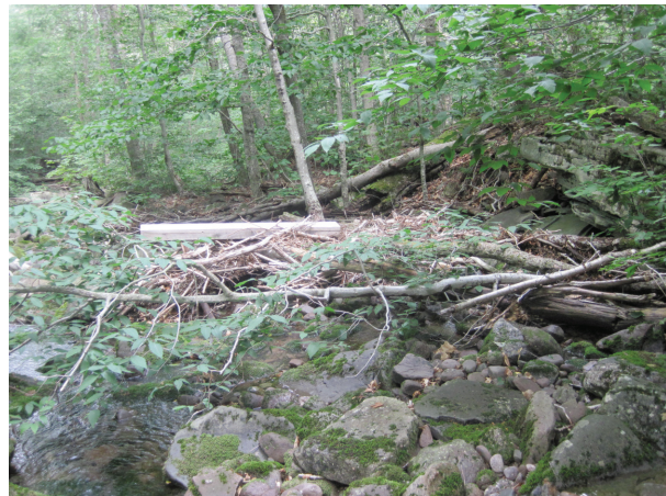
Construction and natural debris causing jam (A548)
