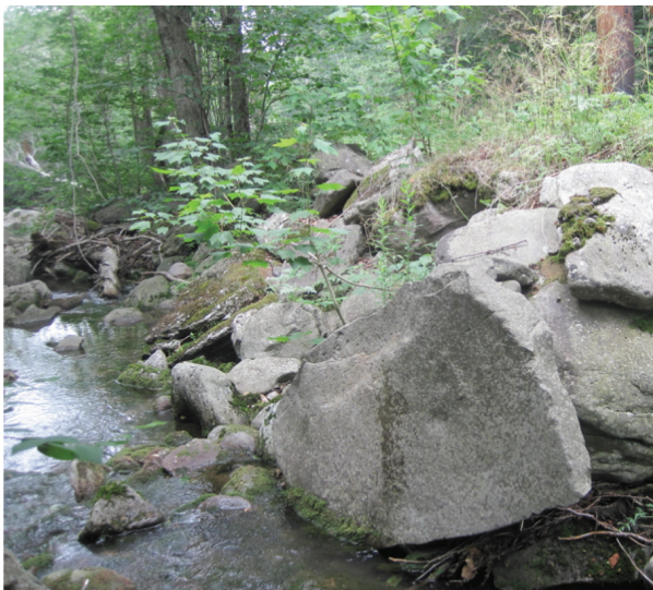
Large boulder revetment that is slumping (A557)
