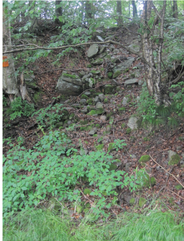
Culvert conveying flow from right valley wall (A601)
