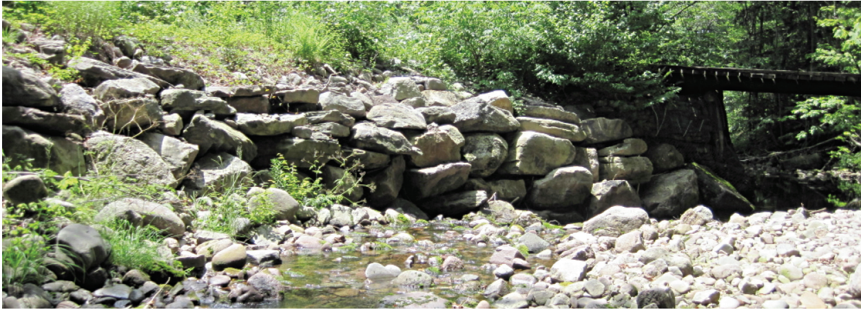
Stacked rock revetment on left bank (A773)
