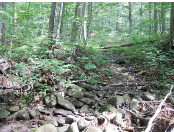
Right floodplain conveying road drainage (A739)
