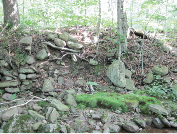
Eroding right bank (A735)
