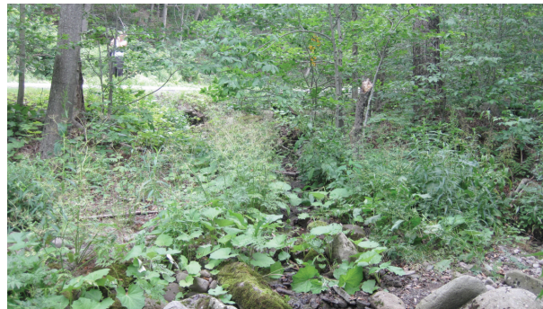
Tributary entering through culvert (B479)
