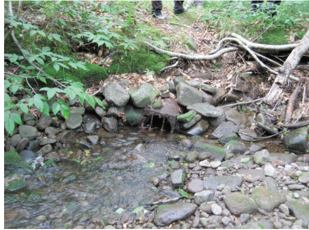
Culvert conveying flow from side channel to pond (A764)
