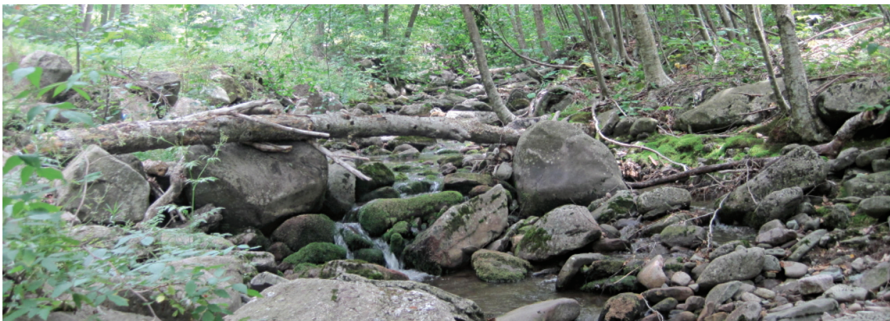
No riparian buffer between revetment and road (A559)
