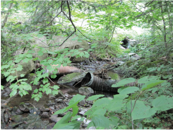
Culvert conveying road drainage (A759)
