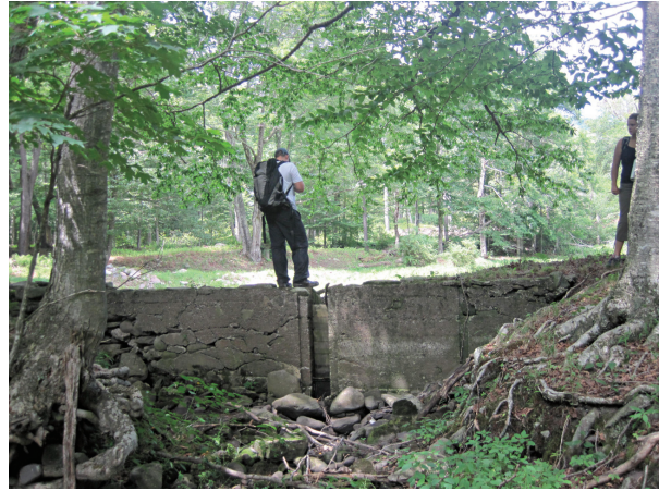
Revetment once used to control drainage from pond (A903)
