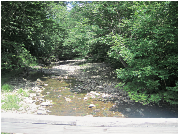
Aggradation upstream of bridge (A909)
