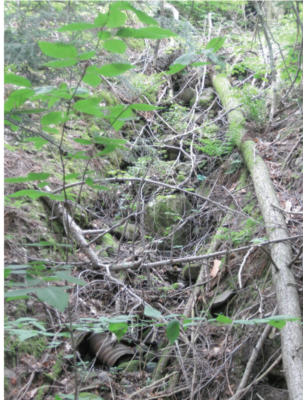
Erosion on right bank (A897)
