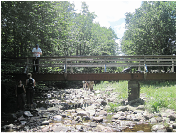
Private footbridge (A907)
