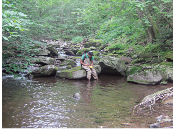
Natural rock weir grade control (B709)
