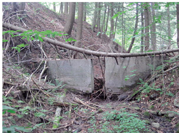
Concrete structure possibly once used to control flow of side channel (A898)
