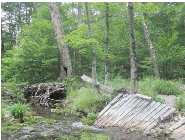
Washed out bridge obstructing flow (A915)
