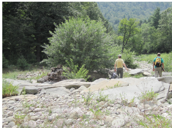
Photo 4.4.3. 6 Check dam on left bank (B533)
