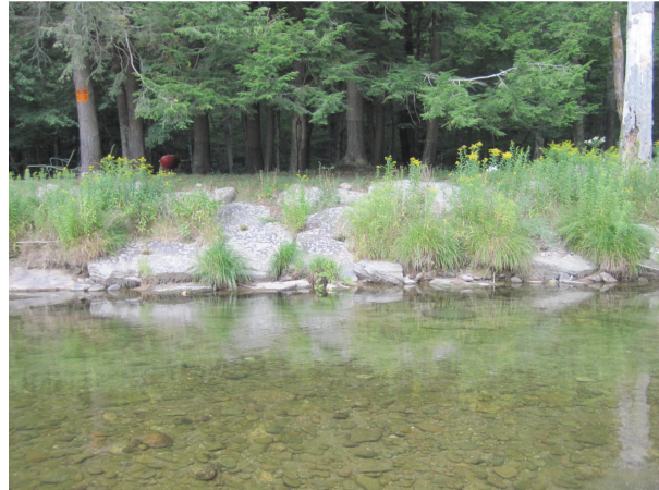
Sloped stone revetment on right bank (A263)
