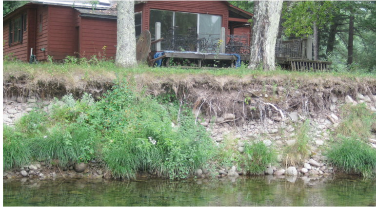
Erosion on left bank (B406)
