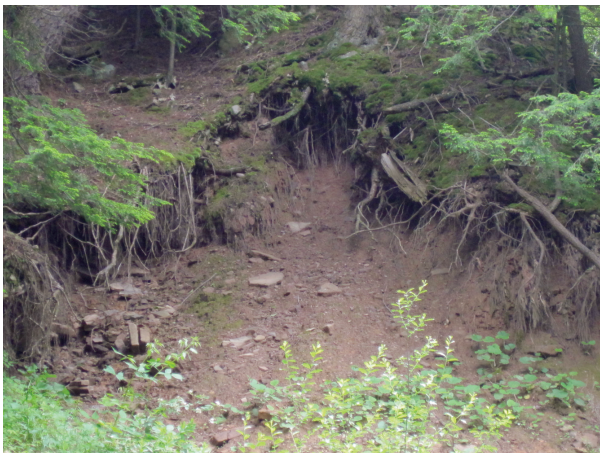
Erosion of right bank (A282)
