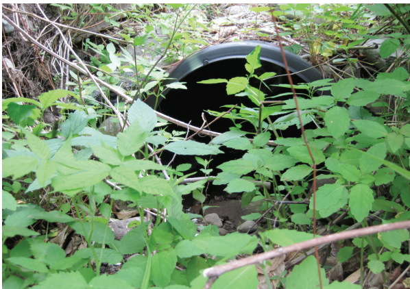
Denning Road culvert pipe (A315)
