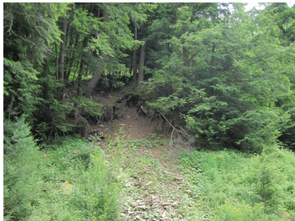
Large rocks deposited at toe of right bank (A284)
