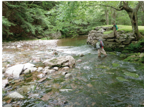
Relict bridge abutments serving as revetment on right and left banks (B171)
