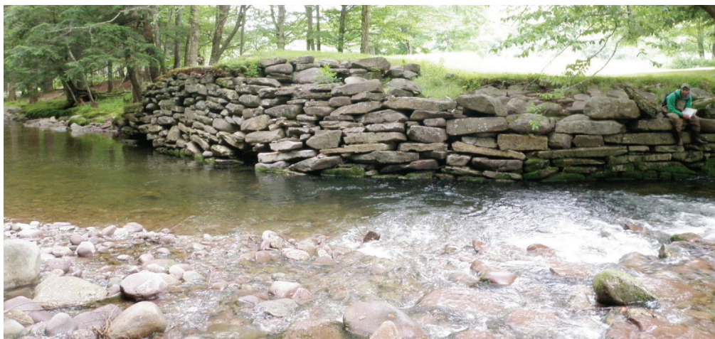
Mowed grass above abutment (B174)
