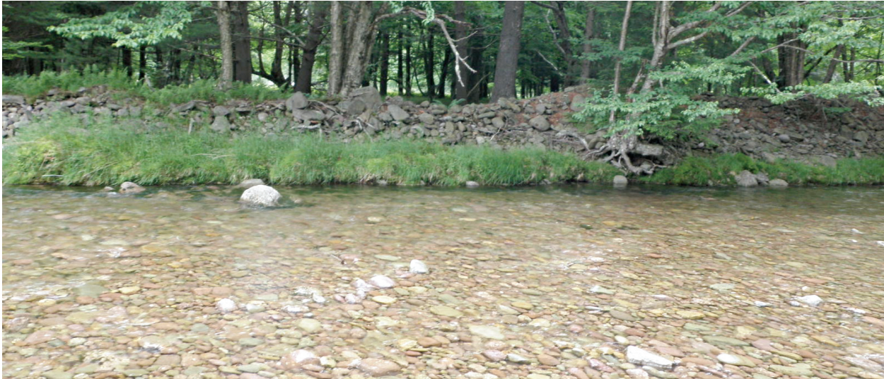
Stone berm on right bank protecting (B208)
