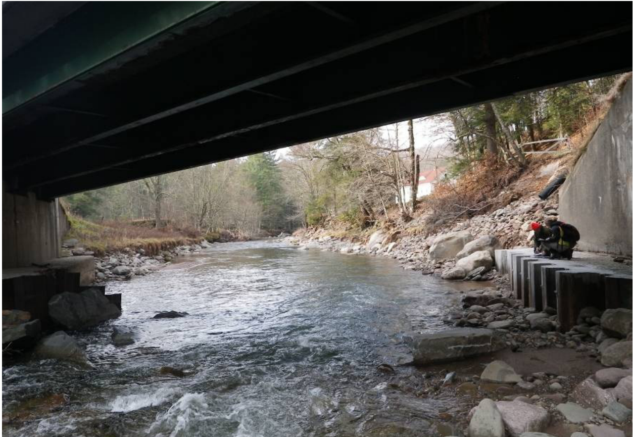
Denning Road bridge—note repair at downstream end of right abutment. Stacked rock revetment has since been installed. (IMG1681)
