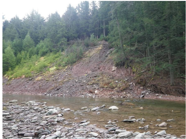
Left bank failure. (IMG1665)
