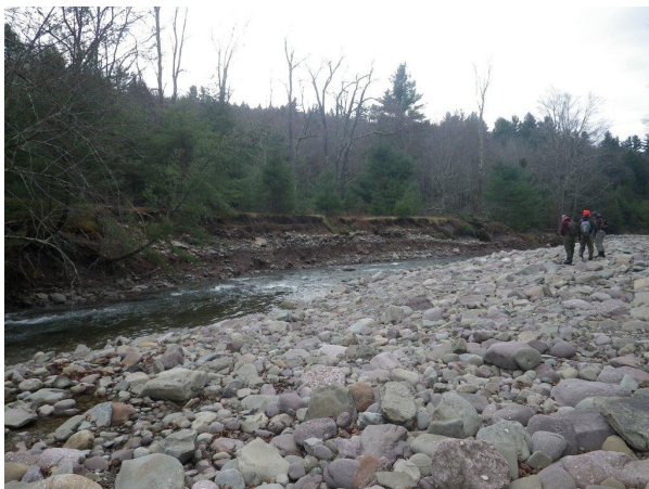
Eroding bank segment on the left bank. (IMGP1654)
