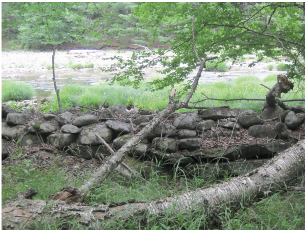
Stacked cobble berm on right bank (B77)
