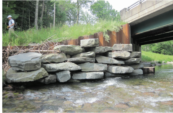
Left bridge abutment with revetment (A116)
