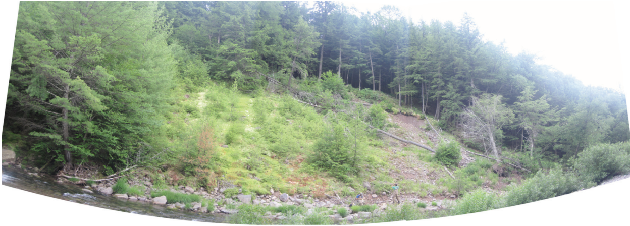
Left bank failure (B101–104)
