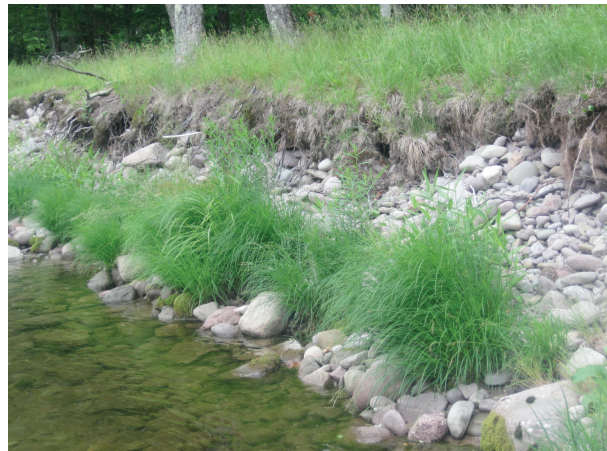
Right bank erosion (A99)
