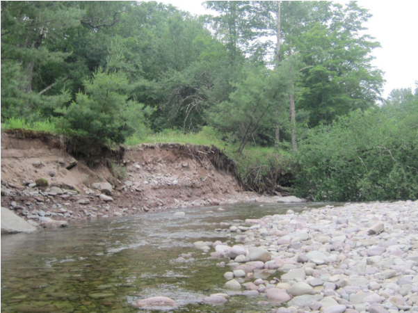
Left bank erosion due to obstruction (B89)
