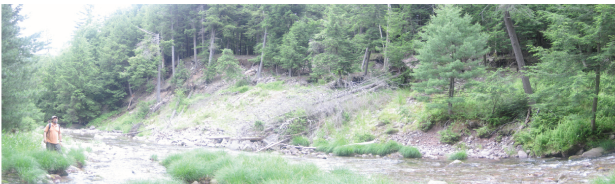
Massive bank failure (A73–75)
