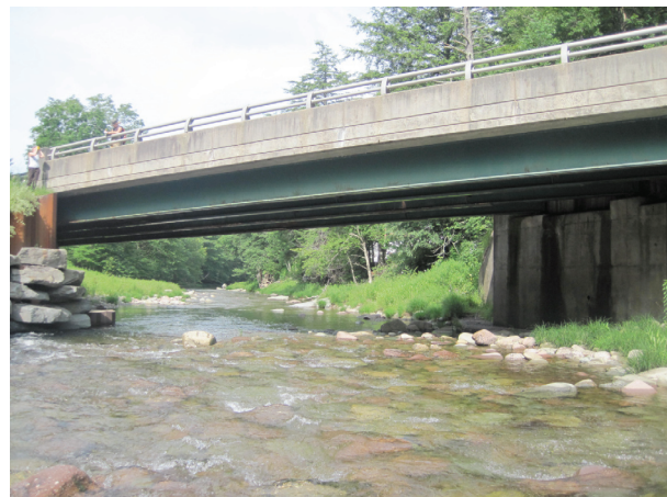
Denning Road bridge (A112)
