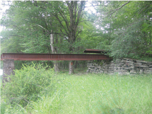
Relict bridge abutment on right bank (A89)
