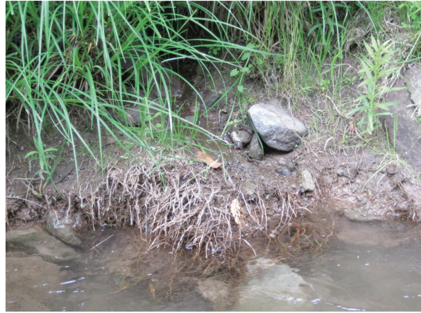
Road drainage entering stream (B71)
