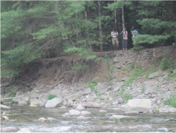
Erosion of right bank (A85)
