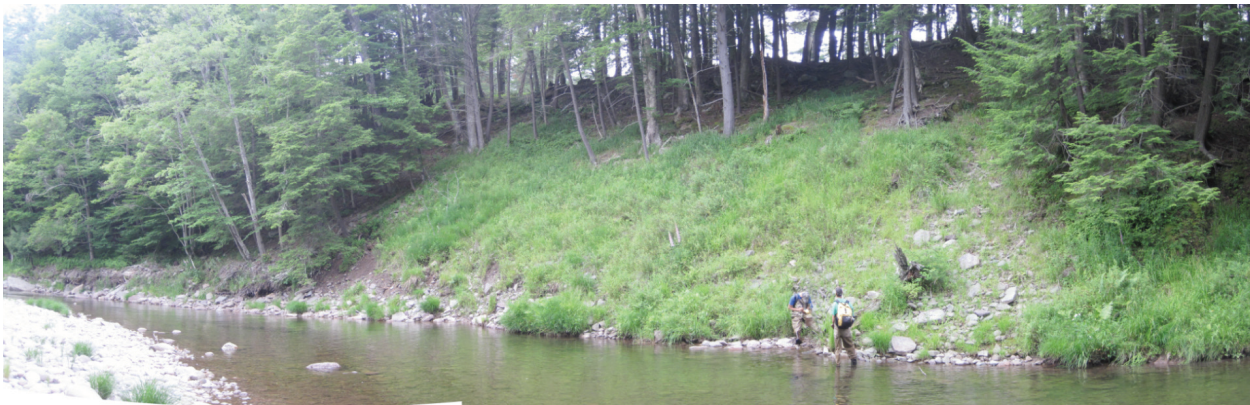
Hill slope failure on right bank (B65–67)
