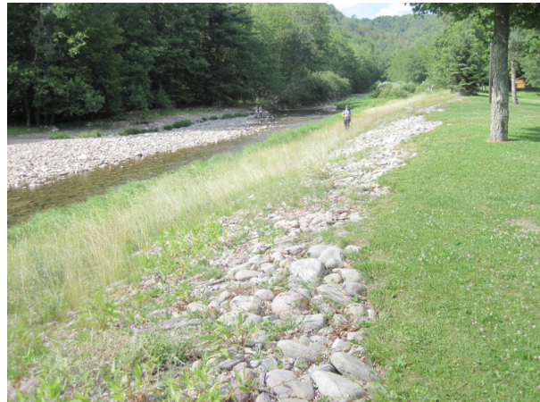
Dumped stone revetment providing temporary stabilization (A430)
