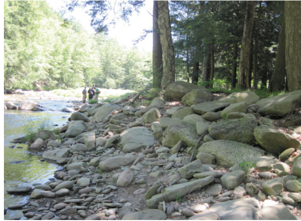
Stacked boulder revetment on left bank (A500)
