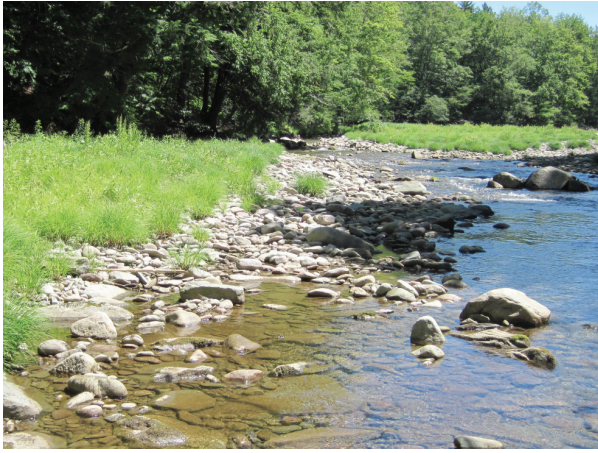
Depositional bar forming across from revetment (B392)
