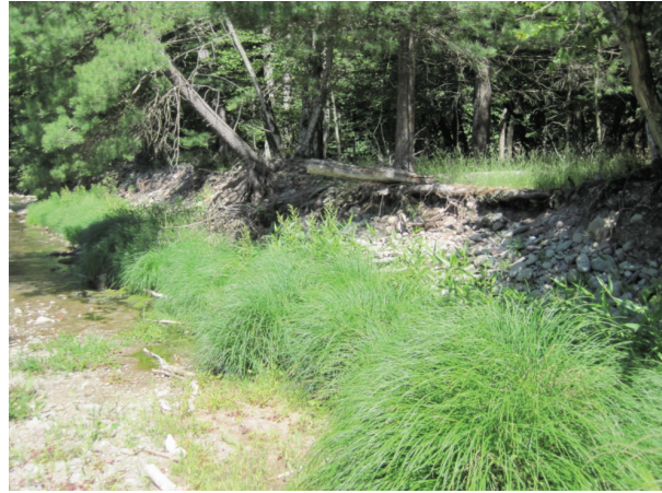
Hydraulic erosion along right bank (A490)
