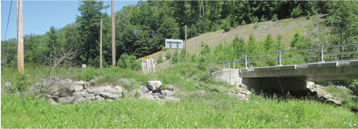
Boulder and cobble sized rip rap on both sides of bridge abutments (B400)
