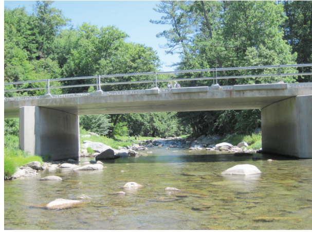
West Branch Road bridge (A507)
