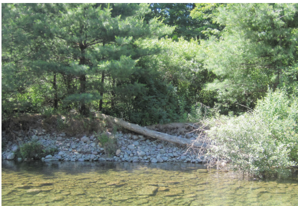
Erosion along left bank (B378)
