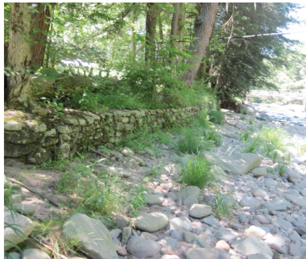
Revetment transitioning to mortared stone wall (A502)
