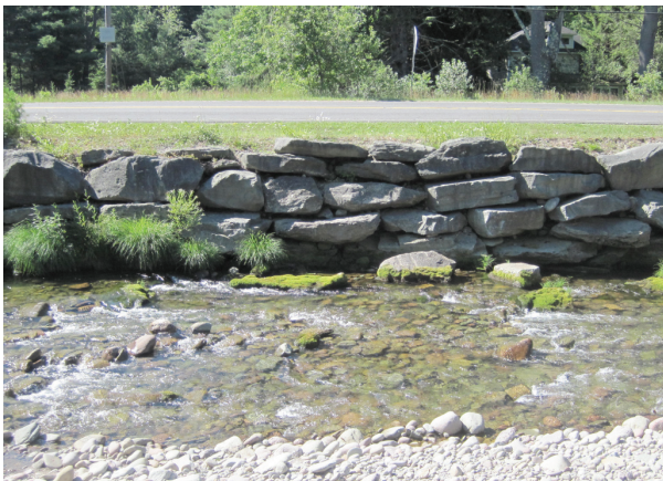
Stacked boulder revetment along left bank protecting road (B349)
