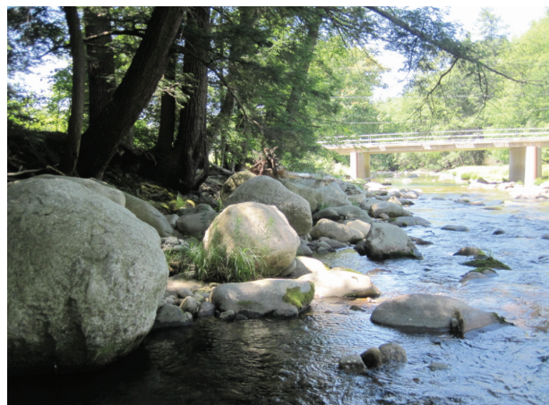
Large boulders placed downstream of stone wall (A504)
