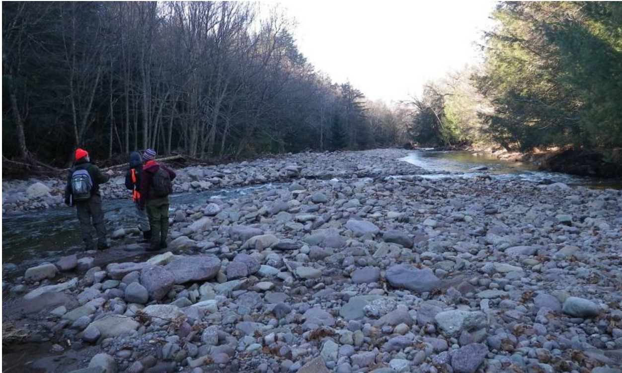
Undersized excavated channel through depositional area. (IMGP1503)
