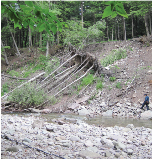
Large failure on right bank (A166)
