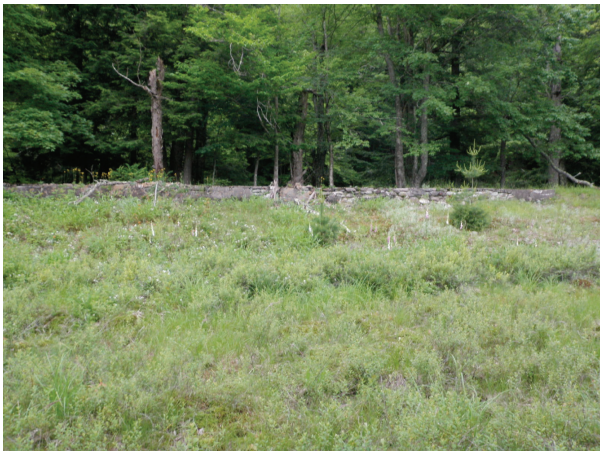
Herbaceous vegetation not providing adequate stabilization (B87)
