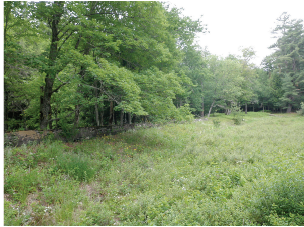
Mortared rock wall revetment on left floodplain (B88)
