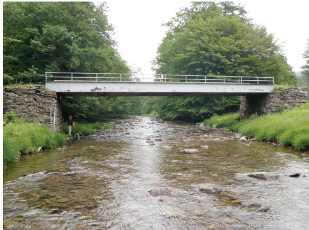
Looking downstream at Frost Valley owned bridge (B92)
