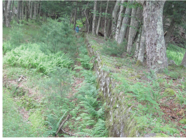
Mortar and stone berm on left bank (A154)
