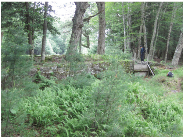
Relict sluice gate (A155)
