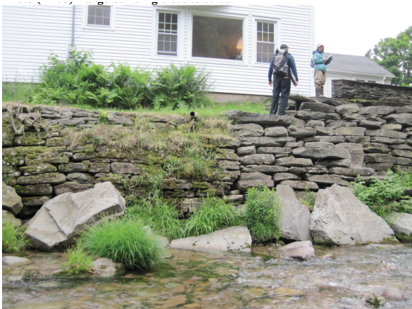
Stacked rock revetment protecting building on left bank (A178)
