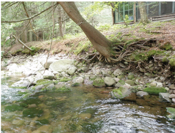
Scour on right bank endangering log home (B78)
