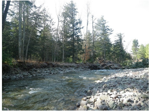
Eroding bank segment and woody debris obstruction. (IMGP1858)
