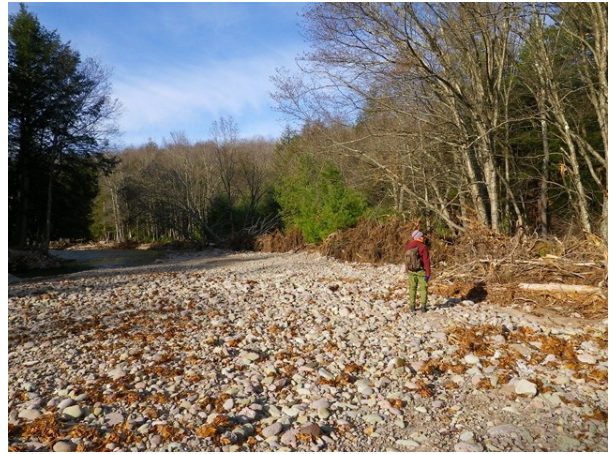
Root wads and large woody debris placed along the tree line behind the cobble point bar. (IMGP1578)
