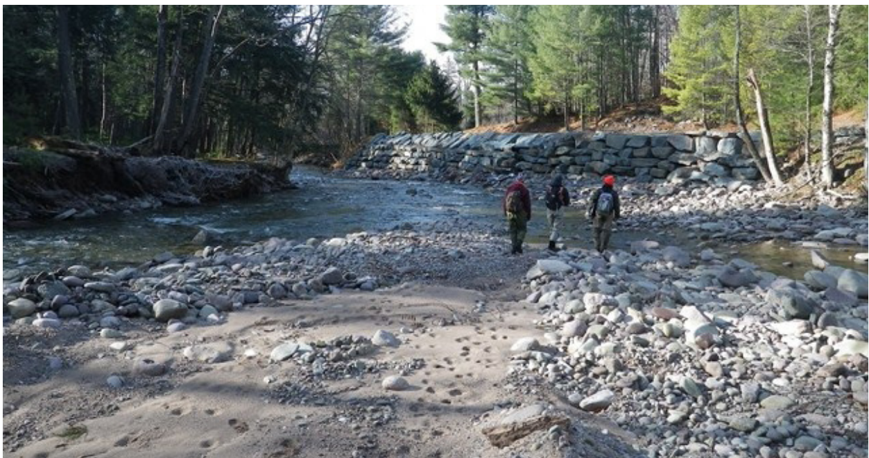
Stacked rock wall on right bank protecting Denning Road. (IMGP1586)
