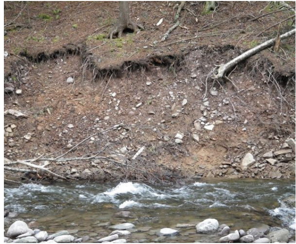
Bank erosion site in need of continued monitoring. (IMG1598)
