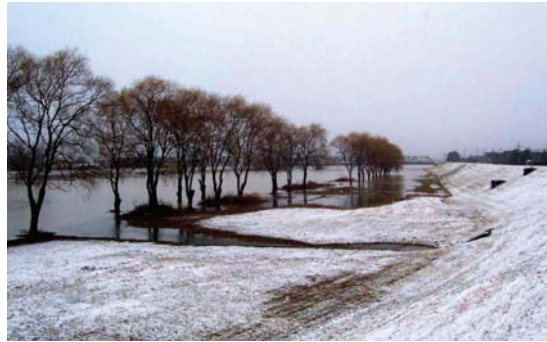
Flood control dike that allows the stream's water to spread out over floodplain, but still provides protection for nearby development (note- this riparian buffer could use enhancement) (Photograph by Scott Rodabaugh, NYSDEC)
