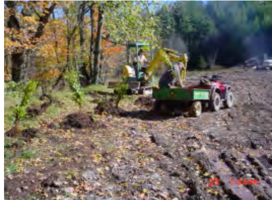
Figure 22: Installation of potted material
