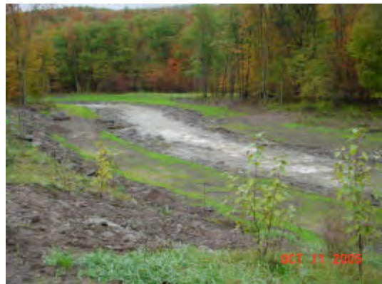
Figure 16: The asbuilt channel after partial bioengineering installation
