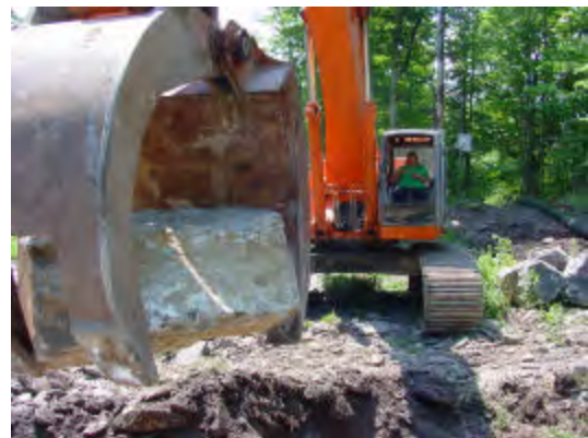
Figure 12: Cross-vane construction
