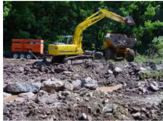
Figure 10: Excavating excess clay from the channel bottom
