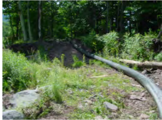
Figure 4: Pipeline used for dewatering
