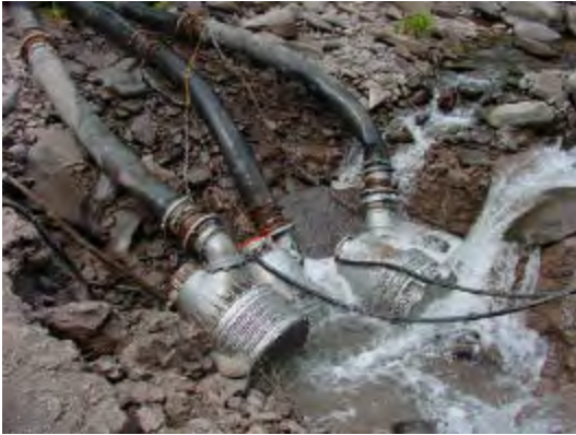
Figure 3: Sump hole for dewatering equipment
