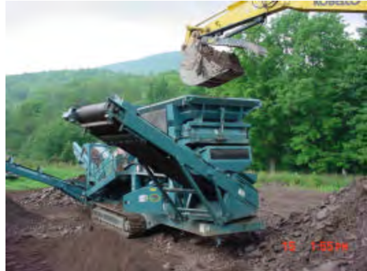
Figure 14: Gravel screen in use
