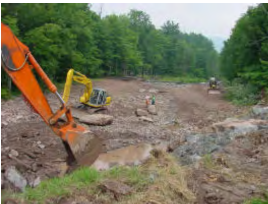
Figure 11: Excavating the design channel
