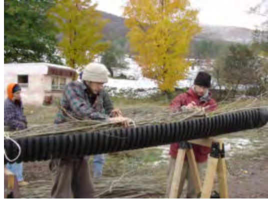
Figure 20: Fascine construction
