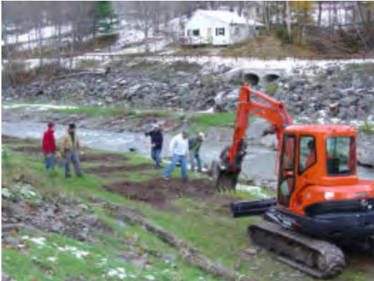
Figure 21: Fascine installation
