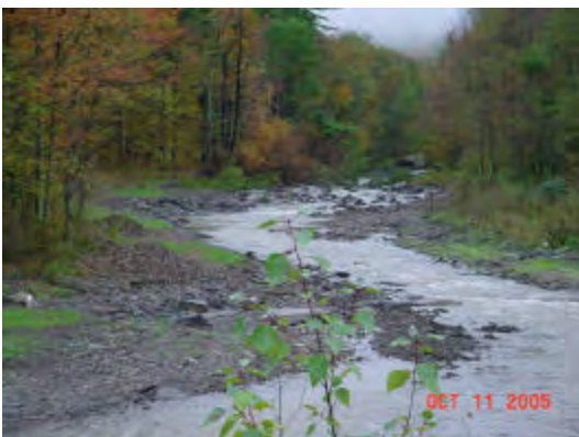
Figure 17: Asbuilt channel after partial bioengineering installation
