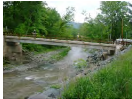
Shoemaker Road bridge, looking downstream
