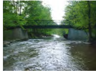
Bridge at RCH Stable
