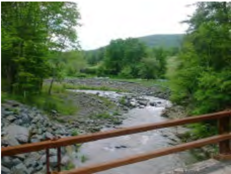
Shoemaker Road bridge, looking upstream
