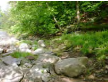
Bank Failure, right
