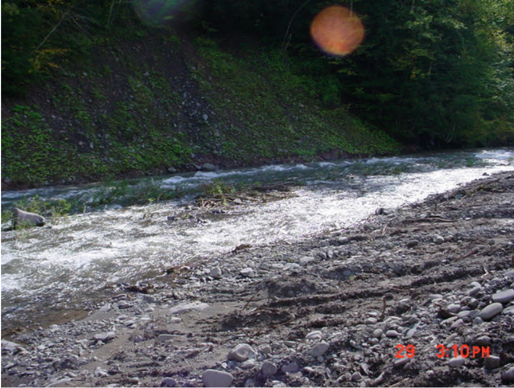
Figure 5: Problem bank near bottom of project area. This section has not been completed. Temporary flood conveyance has been provided on the opposite bank to relieve stress on the problem bank. This area will be treated with temporary seed and mulch.
