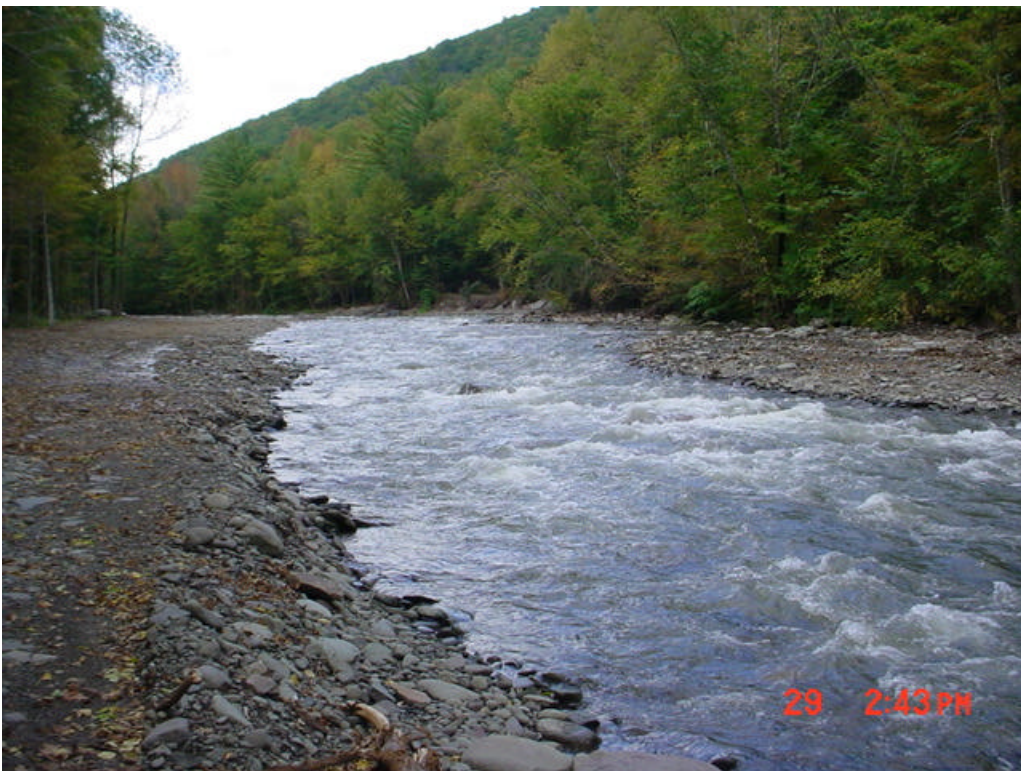
Figure 2: Project area looking upstream from near station 7+50. This section is complete.
