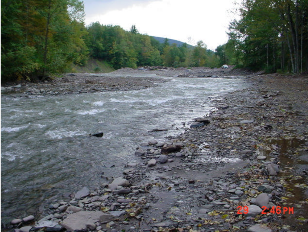
Figure 3: Looking downstream from near station 6+50. Completed section ends at the apex of the bend and flow continues into the incomplete portion of the project area.
