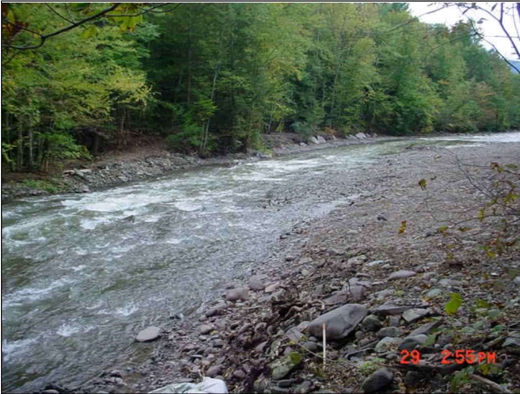
Figure 1: top of project are looking down stream. This section has been completed and is scheduled for bio engineering this fall.
