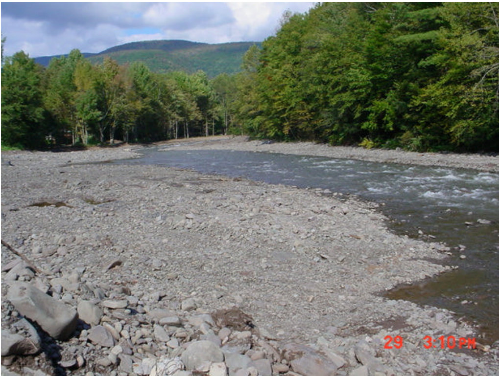
Figure 4: Looking upstream from near station 14+00. this section is incomplete, and scheduled for temporary seeding and mulching.
