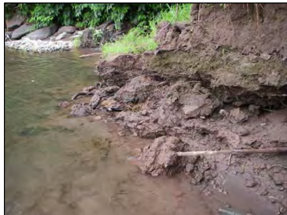
Clay exposure at Station 7600-5850
