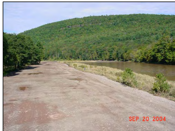
Prattsville flood redemption project post construction
