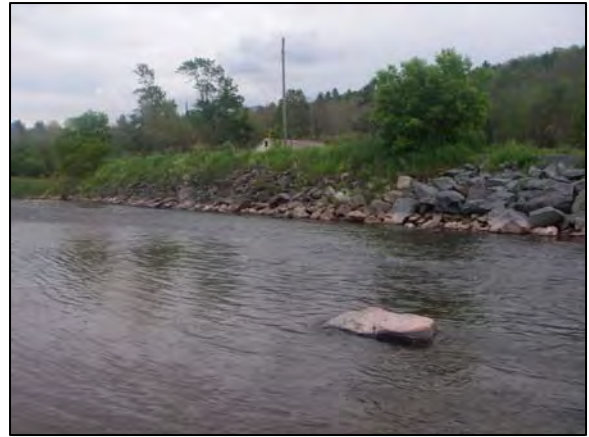
Rip-rap at Station 68300
