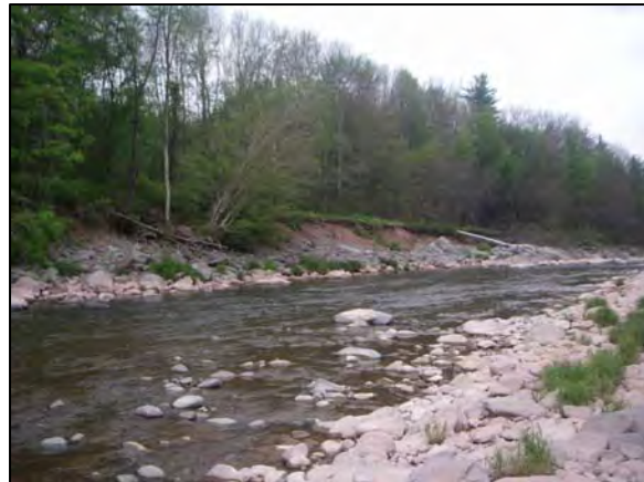
Bank erosion at Station 70450
