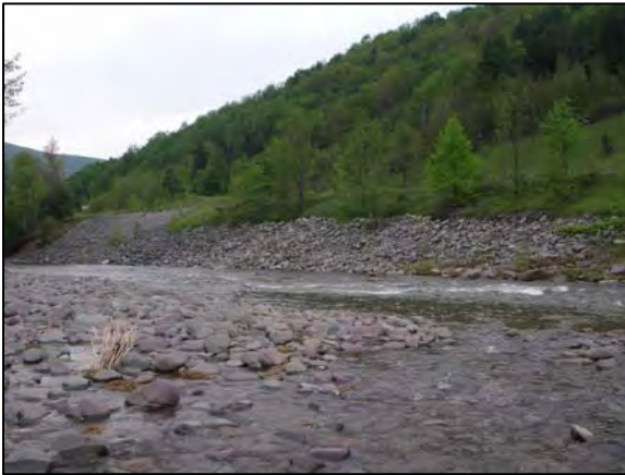
Rip-rap at Station 65200
