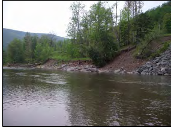
Bank erosion at Station 64580
