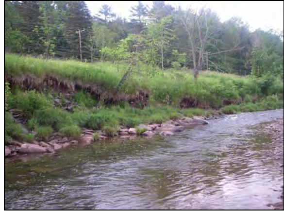
Bank erosion at Station 69050
