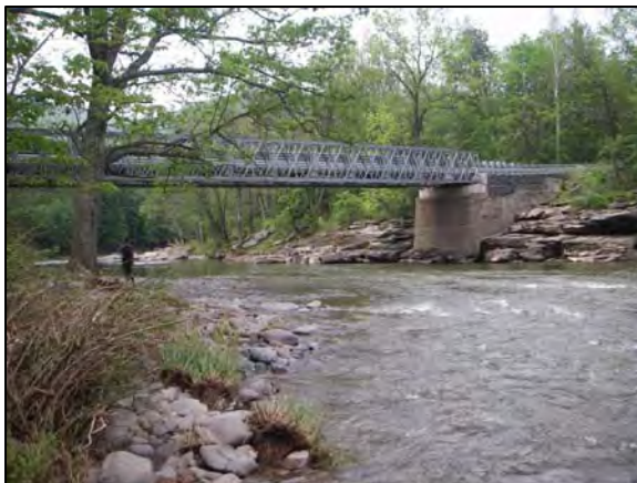
Bridge at Bush Road Station 63446
