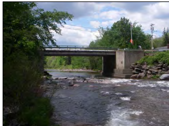
Bridge at Bridge Street – Station 104521
