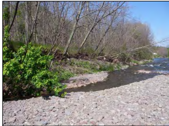
Bank erosion at Station 108100
