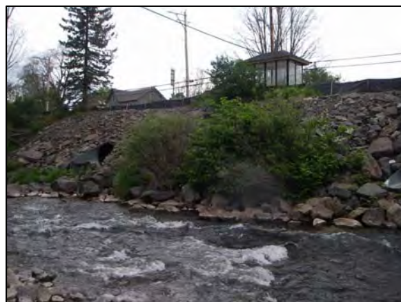
Rip-rap at Station 108500
