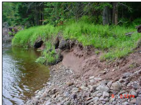
Clay exposure at Station 144700
