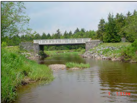
Bridge at Bunny Lane
