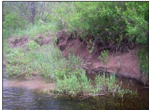
Clay exposure at Station 148740
