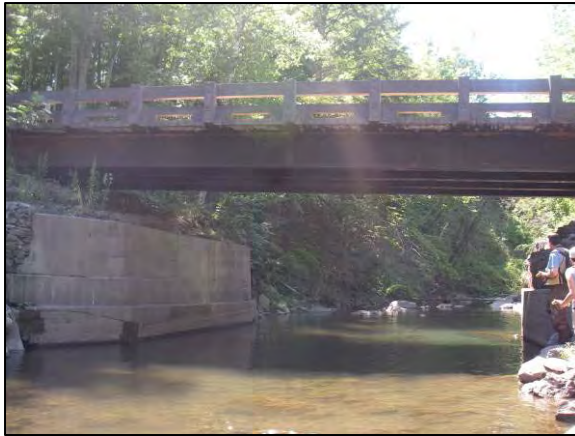
Bridge at Station 8167
