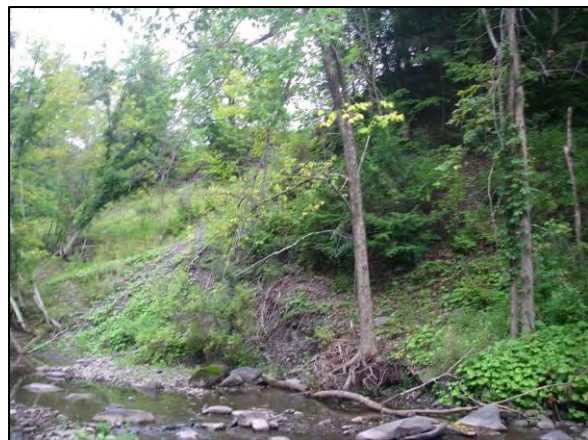
Mass Failure at Stations 8123-7800
