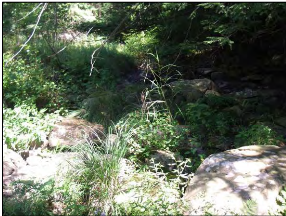
Flood Chute at Station 8426
