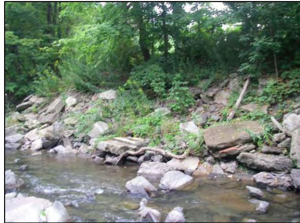
Revetment at Stations 7792-7657
