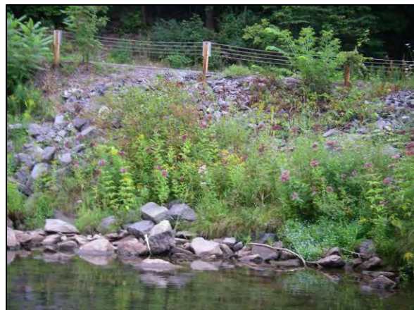
Revetment at Stations 7400-7367
