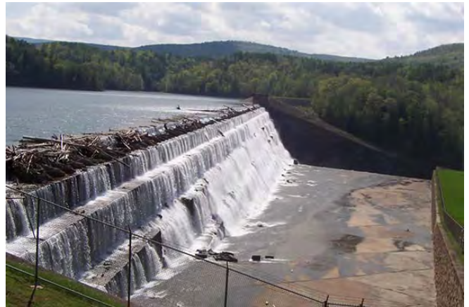
Gilboa Dam at the Schoharie Reservoir www.bearsystems.com
