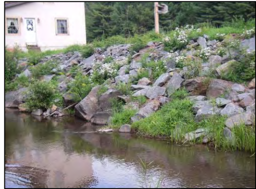
Streamside development and limited riparian vegetation leads to compromised streambanks. This bank has been reinforced with riprap.
