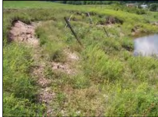
Photo 2.5.4. Hillslope failure in the Manor Kill – notice fence posts moving down with slope.
