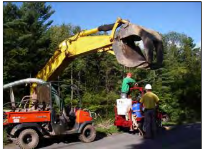
Installation of turbidity control equipment.
