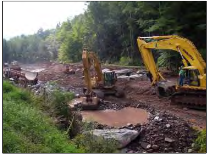
Phase I stream channel excavation.
