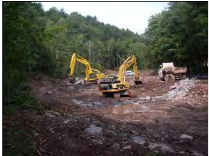
Phase I stream channel excavation.
