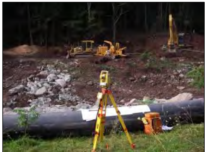
Clearing and grubbing of Phase II.
