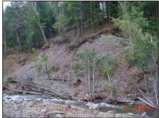
Erosion and failure of high bank.
