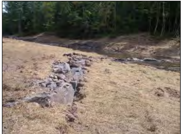
Completed cross vane in upper reach of project.
