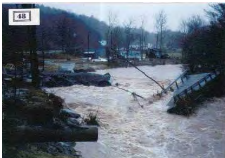
Long Road Bridge during a 1996 flood event.
