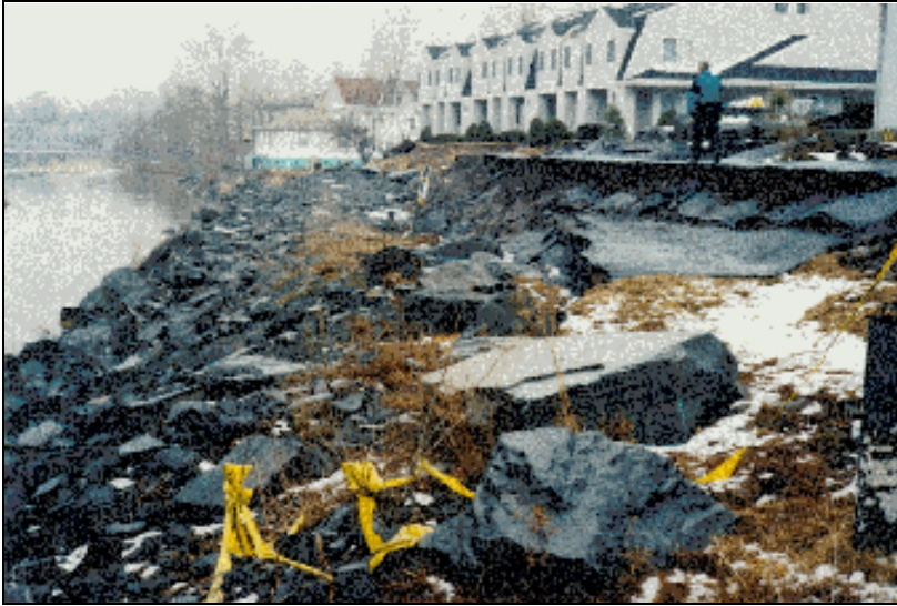
Figure 5.4.1-10 Streambank Failure near Melodywood Condominiums
