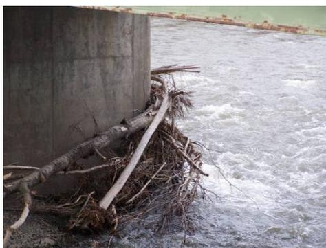
**Photo 4.22: Large Woody Debris (LWD) around bridge pier.**
