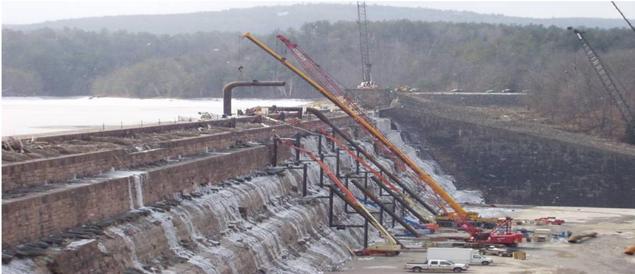
**Photo 2.9: Emergency Reconstruction at the Gilboa Dam on Schoharie Reservoir began in fall of 2005. During the emergency repairs, NYCDEP has operated Shandaken Tunnel at maximum capacity in accordance with the emergency provisions of Part 6 NYCRR § 670.7**
