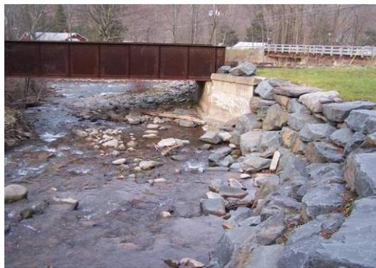
Photo 4.5: Stabilization work upstream bridge.
