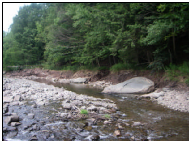
Erosion & clay exposure at Stations 58535 - 58334
