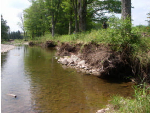
Erosion at Stations 57700 – 577478 Riparian planting site
