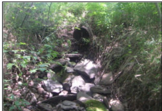
Piped outfall at Station 55864 Photo orientation looking at
