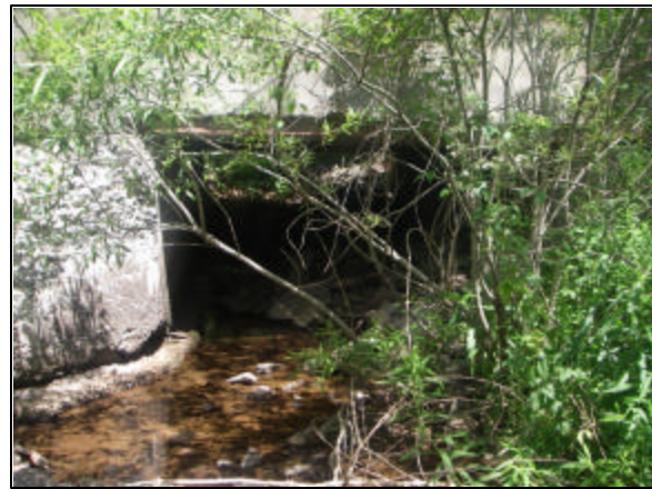
Tributary flow through culvert at Station 55459 photo orientation – looking at
