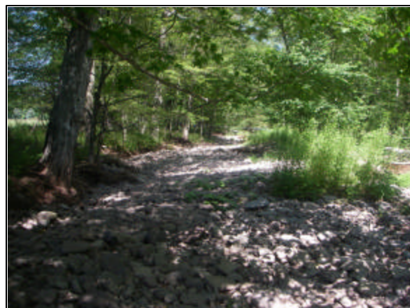
Flood chute at Station 56370
