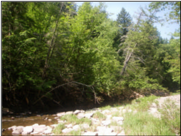
Erosion at Stations 62550 - 61905
