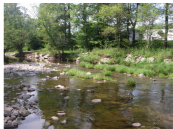
Rip-rap at Stations 51796 - 51200
