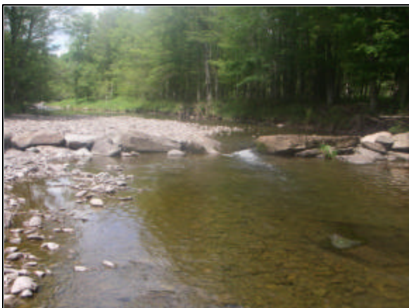
Grade control structure at Station 52653
