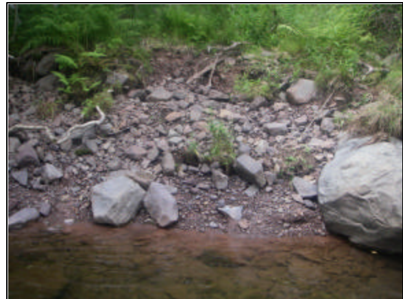
Clay exposure between Stations 53823 – 53754 photo orientation – looking at
