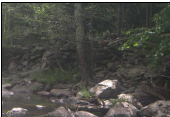
Stacked rock wall at Stations 53332 - 53288
