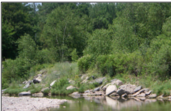
Rip-rap at Stations 59612 - 59066
