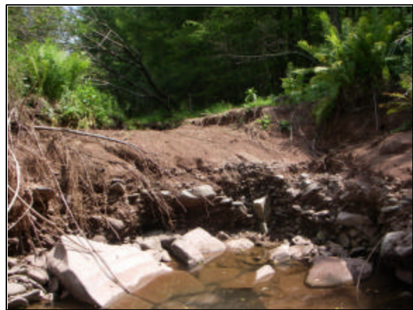
Flood chute and scour hole at Station 57913
