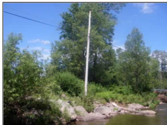
Rip-rap and utility crossing at Station 55120
