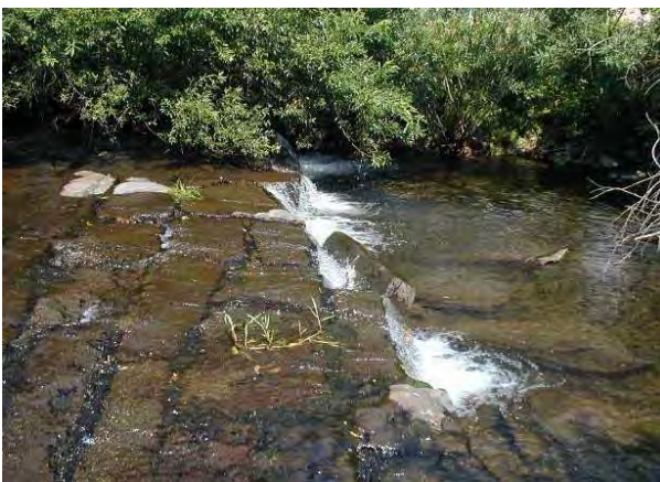
Photo 11. Stone step weir on DEP property at USGS gage.
