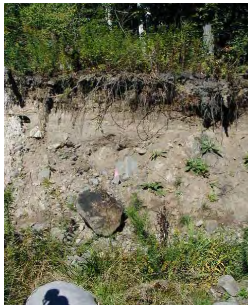
Photo 12. Monitoring cross section, DEP 2, eroded left bank.
