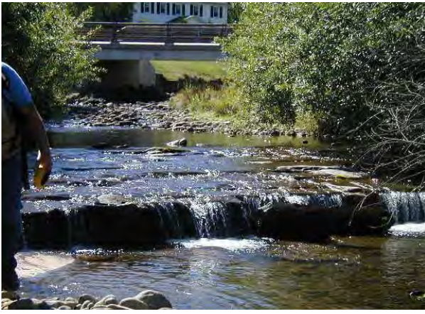
Photo 10. Stone and cement bed-grade control-view looking upstream towards Route 42 Bridge.
