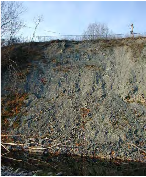
Photo 13. Monitoring cross section, DEP 1, left toe of eroding bank close up of Photo 9, stream flow left to right.
