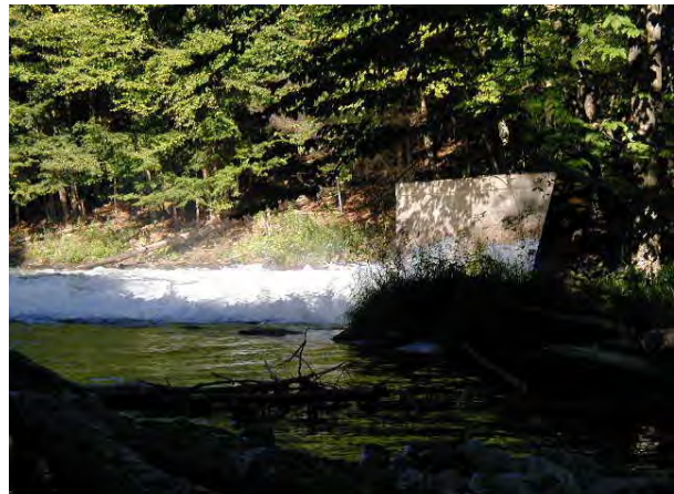
Photo 2. NYC DEP water portal from the Neversink Reservoir, emptying into the Chestnut Creek on the outskirts of Grahamsville, NY.
