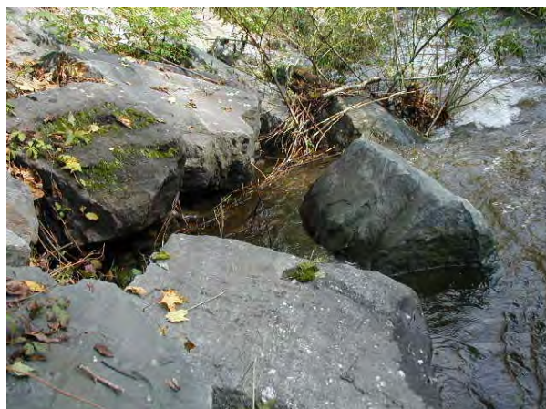
Photo 14. Dislodged riprap in the channel.
