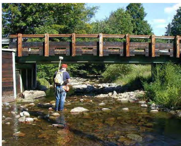
Photo 5. Looking downstream at Clark Road Bridge.
