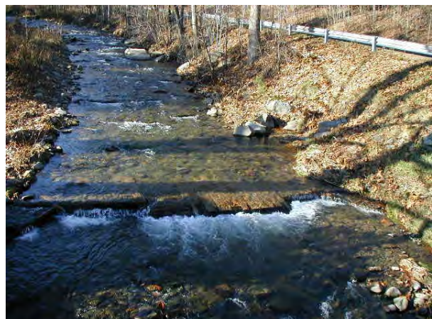
Photo 18. Log sill located just above Covered Bridge.
