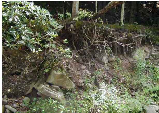
Photo 17. Eroded right bank – view looking upstream near the bottom of MU4.
