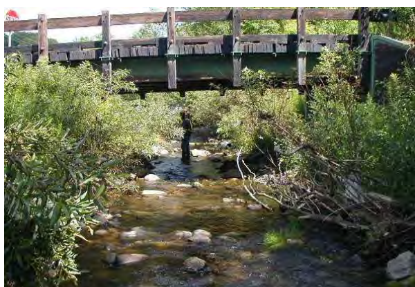
Photo 11. Looking downstream at Kelly Road Bridge.
