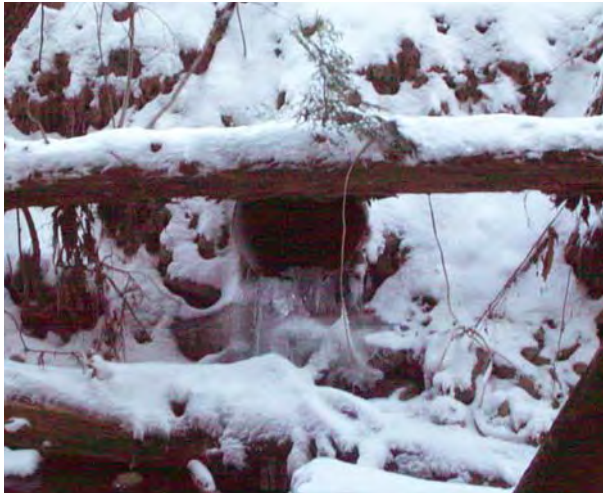
Photo 12. Storm drain outfall behind Zanetti's along Route 55.
