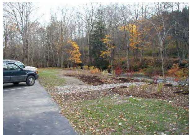
Photo 7. View looking downstream from parking lot. Shows completed swale and planted buffer.
