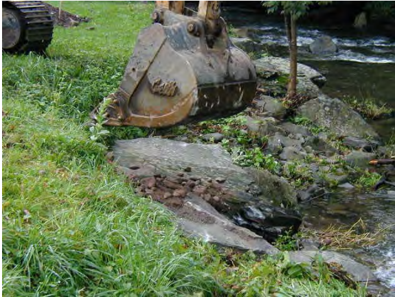
Photo 4. Dislodged riprap removed from the creek and keyed into the eroded bank to create a bankfull bench on September 26, 2003.
