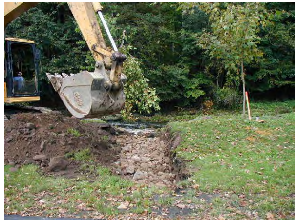
Photo 6. Swale expanded and filled with cobble; September 26, 2003.
