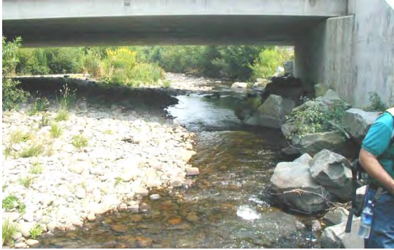
Route 42 bridge Grahamsville, overwidened channel with cobble filling in (right bank) / bridge abutment in main flow of water (left bank).
