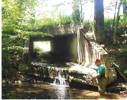
Undercut box culvert and scour pool under Rte 42, on tributary of Red Brook
