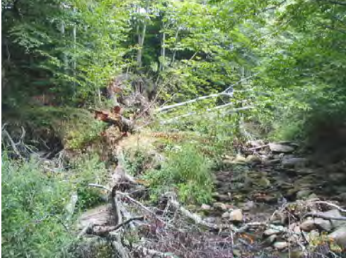
Scott Brook failing bank with fallen trees at Chestnut confluence
