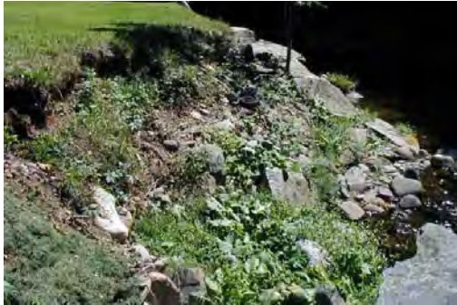
Dislodged riprap behind Town Hall
