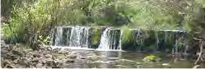
Looking upstream at eroded sewer line structure below Davis Lane Bridge
