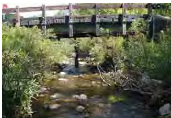
Photo 11. Looking downstream at Kelly Road Bridge.
