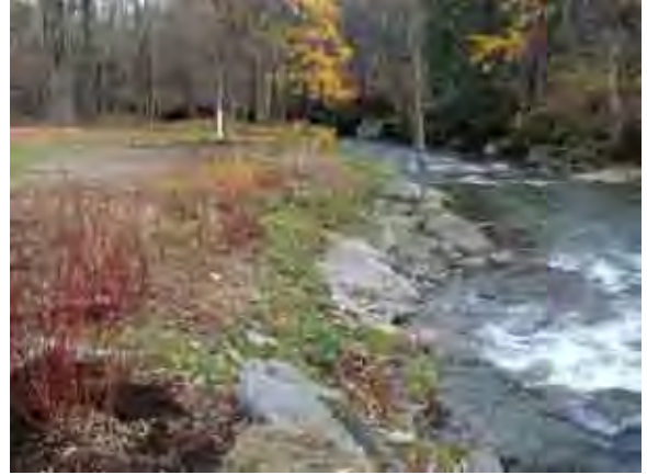
Photo 5. View looking downstream from swale towards stacked rock bankfull bench with new shrubs and native plants.
