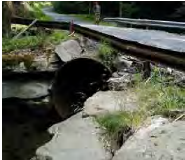
Photo 7. Culvert crossing under Pepacton Hollow Road.
