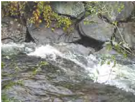
Split channel with riprap on right bank being undermined upstream of covered bridge, within 20' of Route 55
