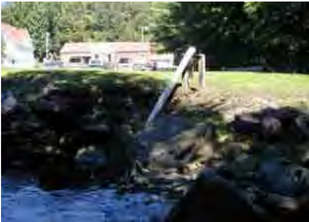
Photo 13. Dry hydrant (out of order, removed) and eroded bank behind Town Hall parking lot-view looking toward left bank & Town Hall from center of stream. (flow left to right)
