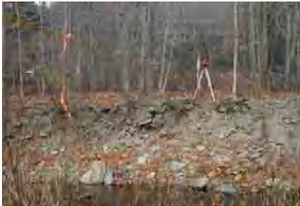
Photo 19. Monitoring cross section 4 at eroded left bank view from right opposite tennis courts at Fair-ground.
