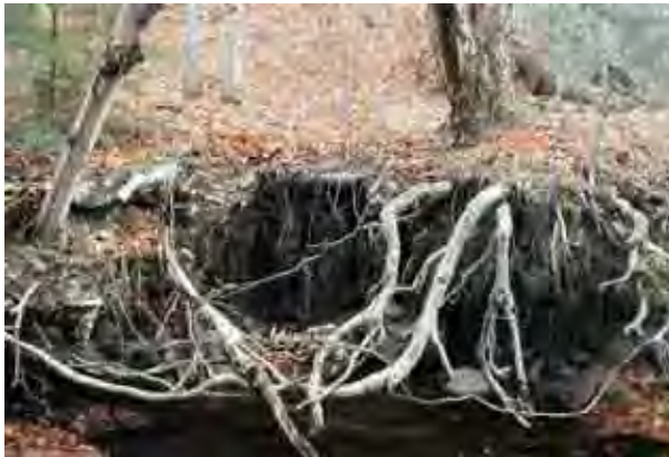
Photo 18. Monitoring cross section 2, left bank above the confluence of Scott Brook with the Mainstem Chestnut Creek. Tree roots and rocks are providing some protection and good habitat.
