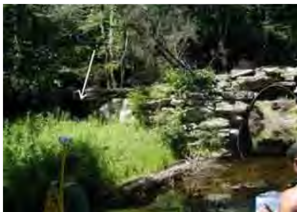
Photo 6. Looking downstream at double culvert Overflow culvert is indicated by white arrow.
