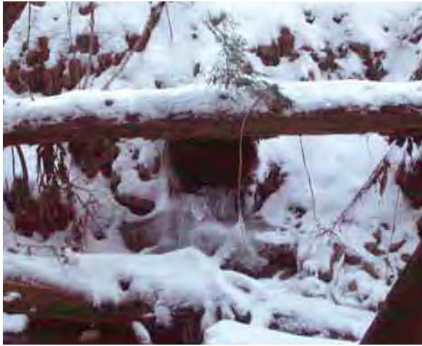
Photo 12. Storm drain outfall behind Zanetti's along Route 55.
