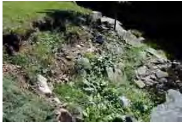
Photo 1. Erosion – left bank behind Town Hall. View looking downstream, dislodged riprap visible in right front corner of photo.
