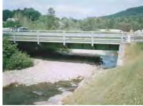
Route 42 bridge Grahamsville, overwidened channel with cobble filling in (right bank) / bridge abutment in main flow of water (left bank).
