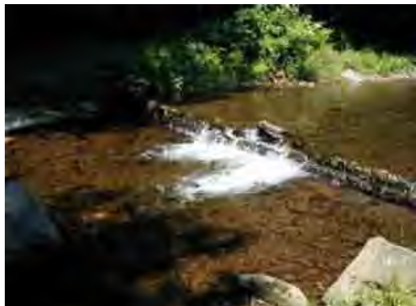
Photo 18. Wood weir behind Town Hall.
