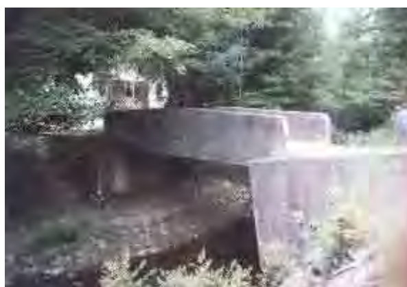
Photo 6. Failing left abutment (on photo right) attached to concrete wall at Mohr's Bridge, stream flow from right to left.
