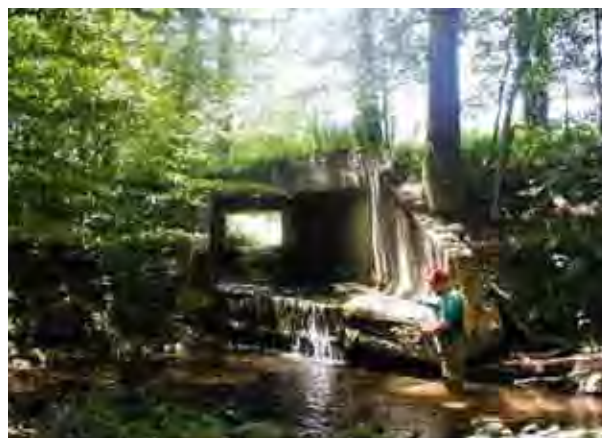
Photo 7. View from mid channel looking upstream. Scour pool at outlet of Route 42 box culvert. Eroding right bank 10' high.
