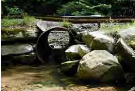
Looking upstream at culvert under Pepacton Hollow Rd.
