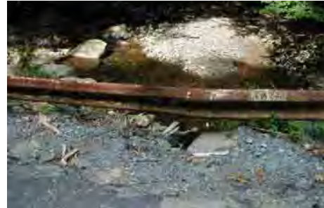
Erosion under guardrail above outlet end of culvert (2001)
