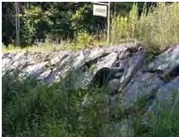
Photo 10. rip-rap along left bank and Rt. 55 with 2' diameter culvert from the road – below Mohr's bridge.
