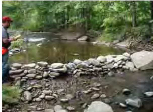
Photo 16. Rock check dam, between Clark Road Bridge and Hilltop Road Bridge.
