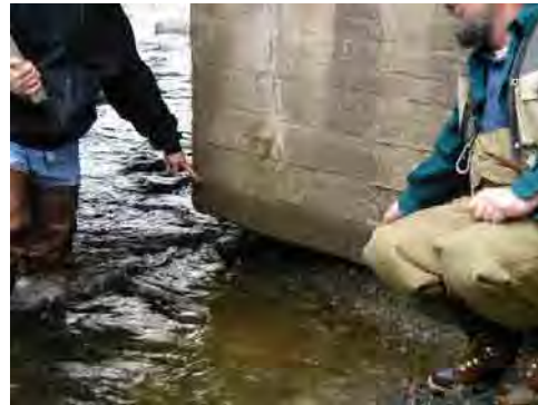
Crack in upstream right wing wall of Covered Bridge and 14 inch undercut
