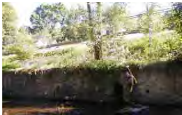
Photo 16. Concrete wall with box culvert along Route 55 between River Road and Fire House.
