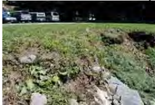
Eroded left bank and lack of vegetation behind Town Hall
