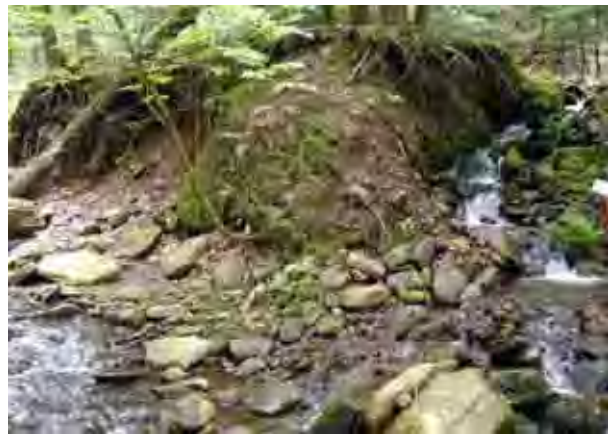
Photo 3. View looking upstream at left bank and confluence with another tributary downstream of Photo 2 (on right side of the photo) that flows under Camp Road. Significant erosion.
