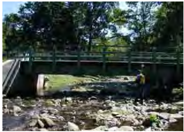
Photo 8. Looking downstream at River Road Bridge, just above Town Hall. Note the cobbles that are deposited upstream of the bridge in the foreground of the photo.
