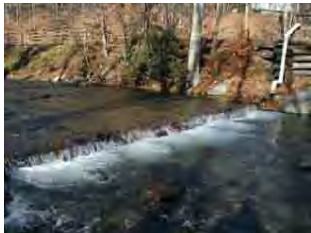
Photo 17. Just below Covered Bridge MU5, Wood Weir serving dry hydrant in downstream MU (see MU6 for more detail).
