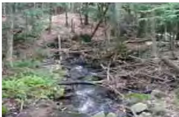
Photo 15. Looking downstream at major debris jam on right branch of split channel.
