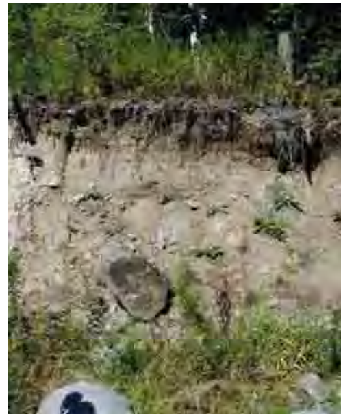
Photo 12. Monitoring cross section, DEP 2, eroded left bank.
