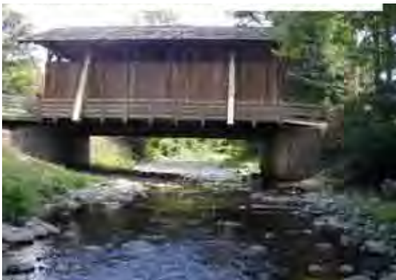
Photo 1. Looking downstream upstream at the historical Covered Bridge at the Town of Neversink, Agricultural Society Fairgrounds along Route 55, at bottom MU 5.
