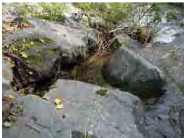
Photo 14. Dislodged riprap in the channel.
