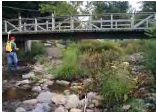
Photo 10. View looking downstream at private crossing below Slater Rd. Channel is split with a center island. The banks and island are well-vegetated with willows, but stream seems to be choked into the right bank.
