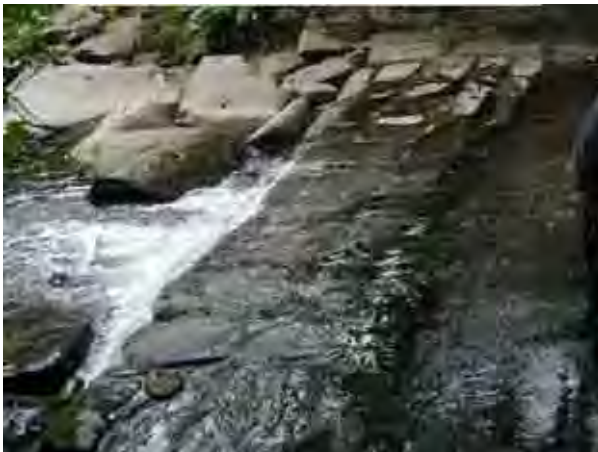
Photo 11. Rock and cement bed/elevation control – looking toward right bank below Clark Road Bridge.
