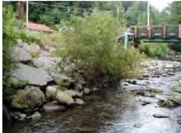
Photo 13. Rip-rap on right bank below Clark Rd. Bridge – view looking upstream at end of bridge opposite from Route 55.
