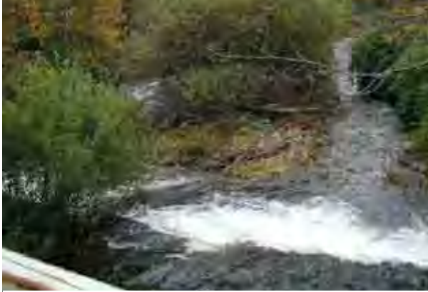
Photo 10. Looking downstream from top of Davis Lane Bridge at split channel below grade control at high flow. Right channel dry in 2001 at low flow. Center bar with cobbles and willow can be seen.
