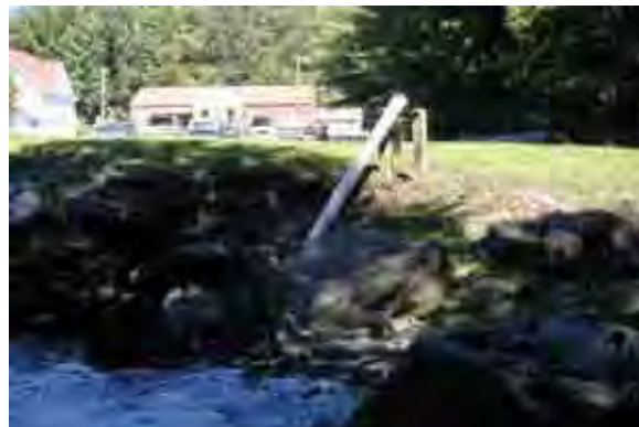
Photo 3. Dry hydrant behind Town Hall parking lot. View looking toward left bank from center of stream.
