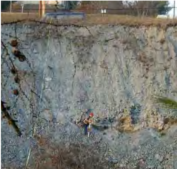
Photo 4. View of eroded left bank on DEP property. Material undercut and slumping.
