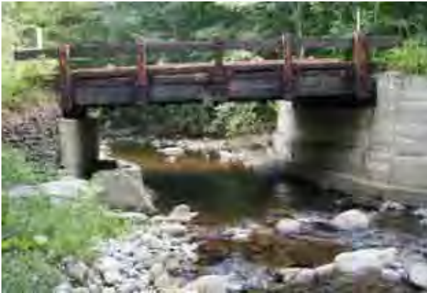
Photo 8. View looking downstream at Hilltop Road Bridge, gabion revetment can be seen on left of photo.
