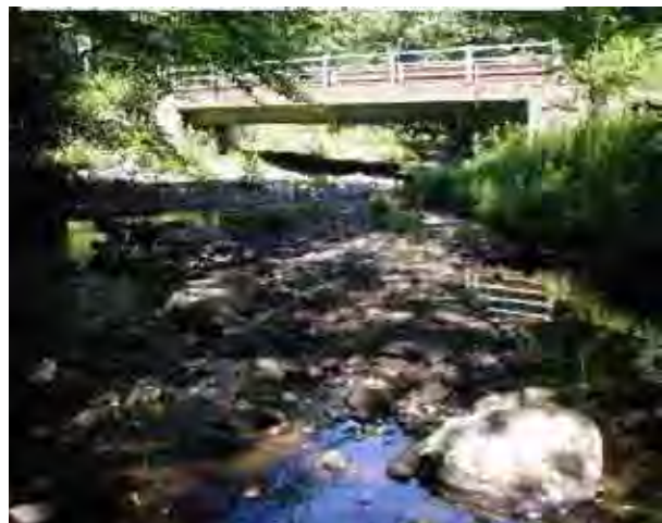
Photo 4. View looking at South Hill Road Bridge.
