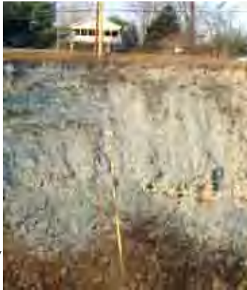
Looking at eroding bank with BEHI XS
