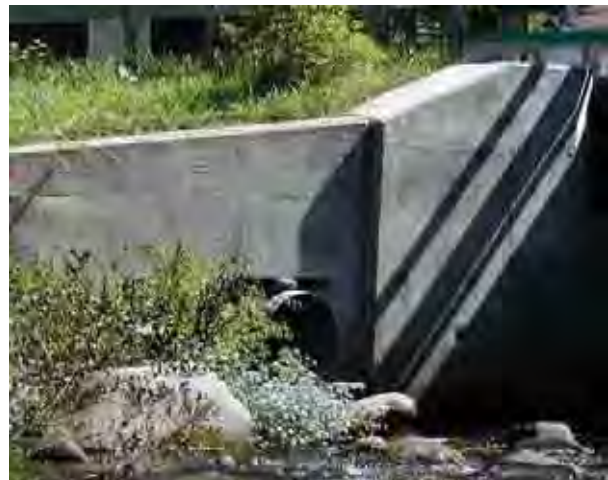
Photo 14. Culvert in left bank abutment on upstream side of River Road Bridge, view looking downstream from the center of the stream.
