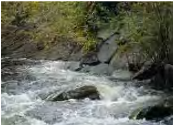
Photo 12. Left channel riprap looking upstream several hundred feet above covered bridge opposite fairgrounds.
