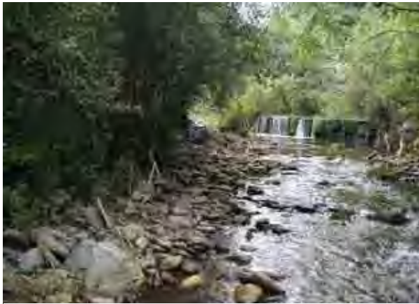
Photo 11. Looking upstream towards Davis Lane Bridge concrete grade control structure over sewer line.
