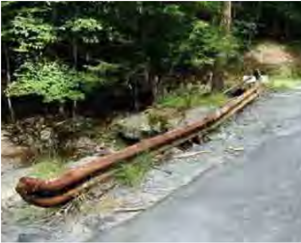
Photo 4. Recent storms have overtopped the road at this culvert, causing damage to the road. FEMA funding replaced guardrail seen in photo, 2002.
