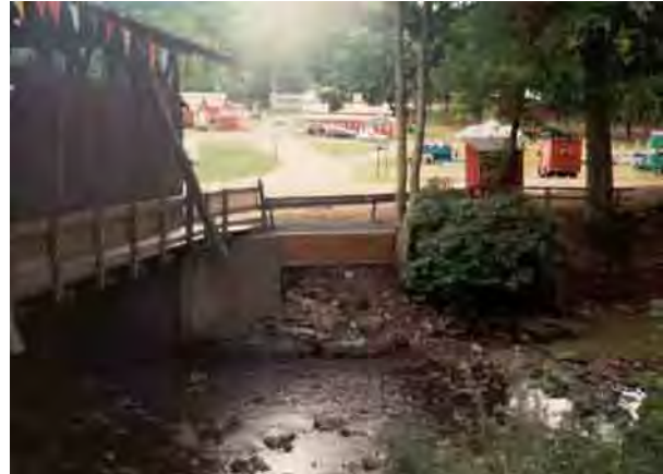
Photo 9. Looking upstream right bank Covered Bridge and Fairgrounds. Archive photo obtained from NYS DEC of repair work conducted on wingwall scour in 1991.
