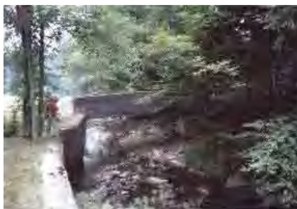
Photo 7. Looking downstream at concrete wall on left bank tied into edge of Route 55 and Mohr's Bridge.
