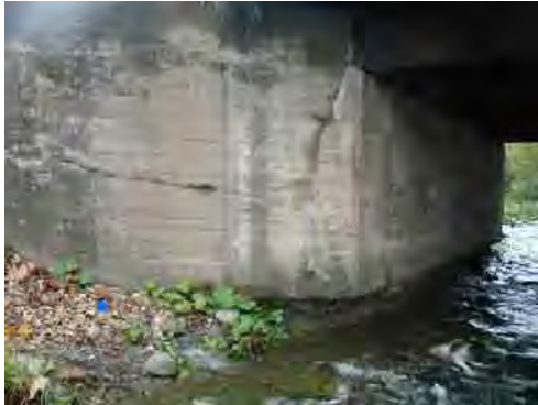
Crack in downstream right wing wall of Covered Bridge
