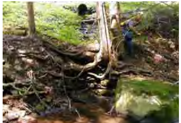
Photo 8. Looking at culvert (top of photo) under Pepacton Hollow Rd. right stream bank, stream flow right to left.
