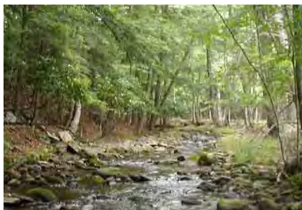
Photo 19. View looking upstream from inlet end of culvert under Pepacton Hollow Road at intersection with Brenner Road.
