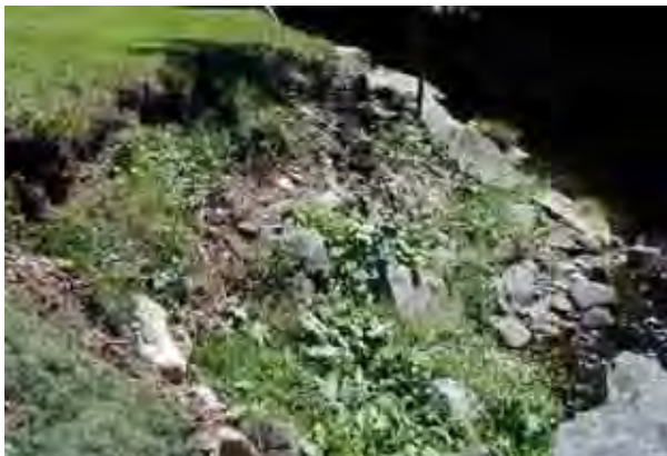
Photo 17. Dislodged riprap at left bank behind Town Hall parking lot-view looking downstream with dry hydrant partially visible in the background.
