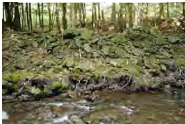
Photo 10. Looking at undercut right bank and berm, stream flow left to right.
