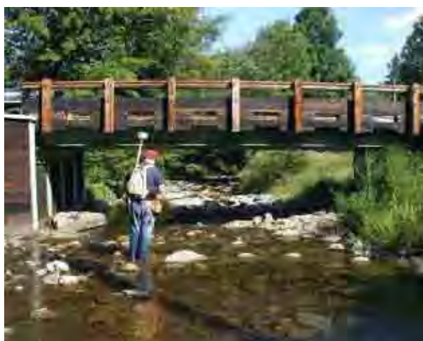
Photo 5. Looking downstream at Clark Road Bridge.
