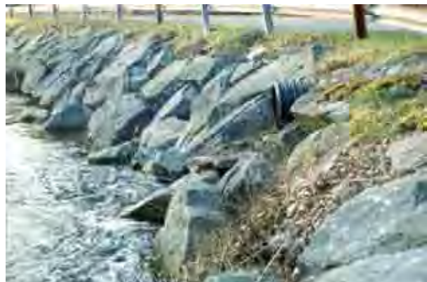
Photo 12. Looking downstream at rip rap along sharp curve and culvert on right bank, along River Road upstream of bridge. Flow hits directly into bank near culvert.
