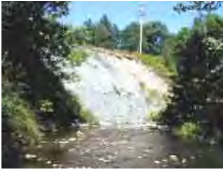
Looking downstream at high eroding bank DEP property
