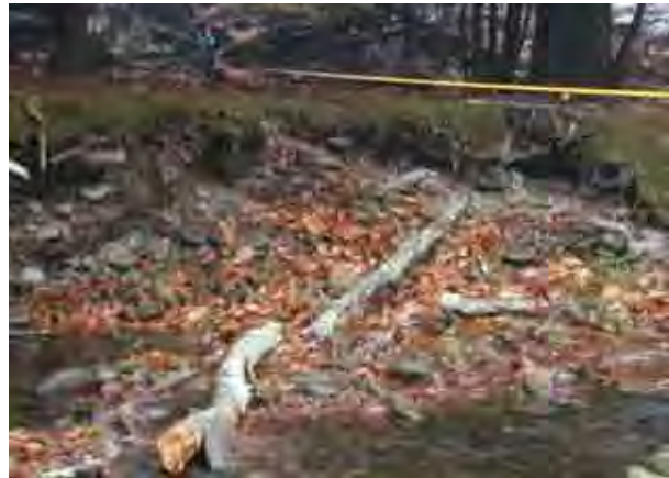
Photo 21. Monitoring cross section 6, approximately 200' eroded right bank, downstream of monitoring cross section 5.
