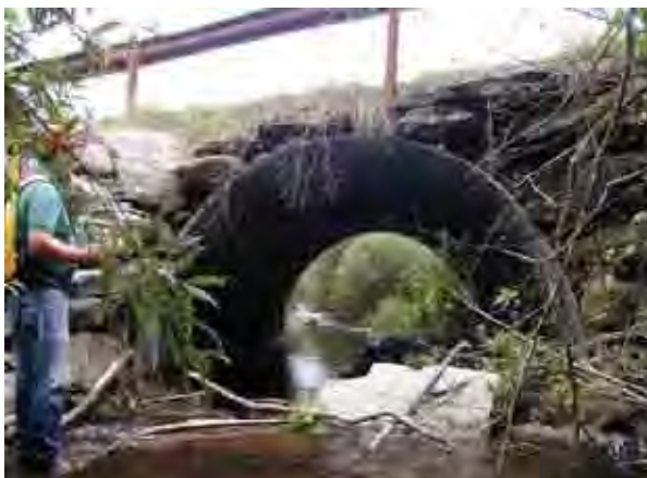
Photo 9. View looking downstream at inlet of culvert under Slater Road.
