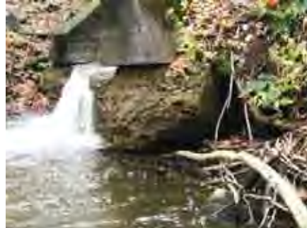
Undercut box culvert and scour pool under Rte 42, on tributary of Red Brook
