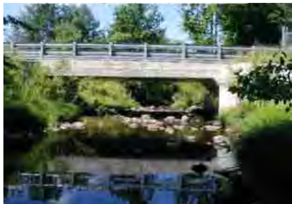
Photo 3. DEP bridge over Red Brook.
