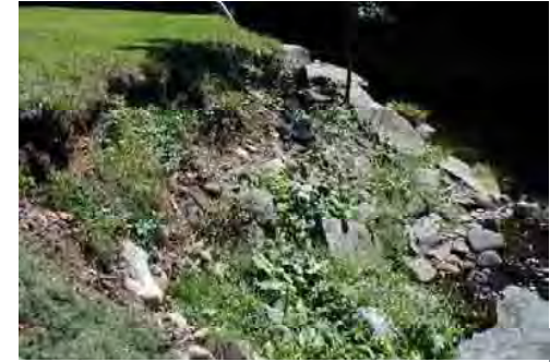
Erosion-left bank behind Town Hall parking lot view looking downstream with dry hydrant visible in the background
