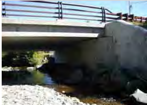
Photo 1. View looking downstream at Route 42 Bridge, cobble bar under bridge with main channel flowing into right abutment armed with riprap.
