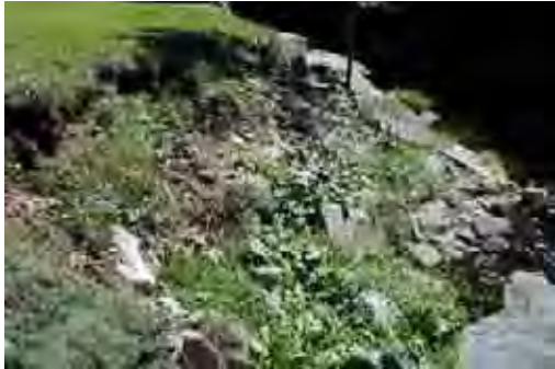
Dislodged riprap behind Town Hall
