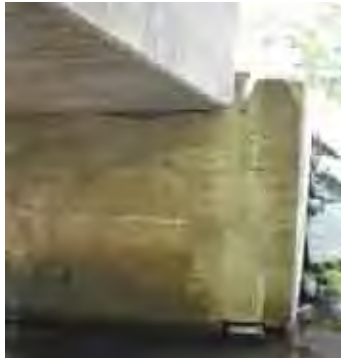
Concrete crib wall along Rte. 55 attached to failing abutment
