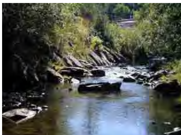
Photo 9. End of rip-rap on right bank, downstream of Route 42 Bridge – on DEP property – view looking upstream from the center of the stream.
