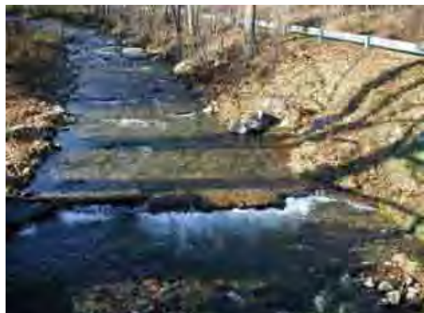
Photo 18. Log sill located just above Covered Bridge.
