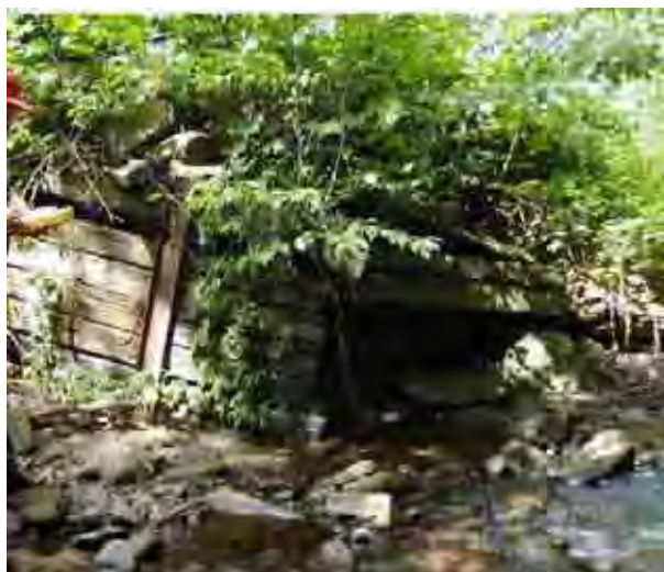
Photo 14. Beginning of log crib wall on left bank view from right bank near bottom of MU4, before the entry of the Claryville Road tributary.
