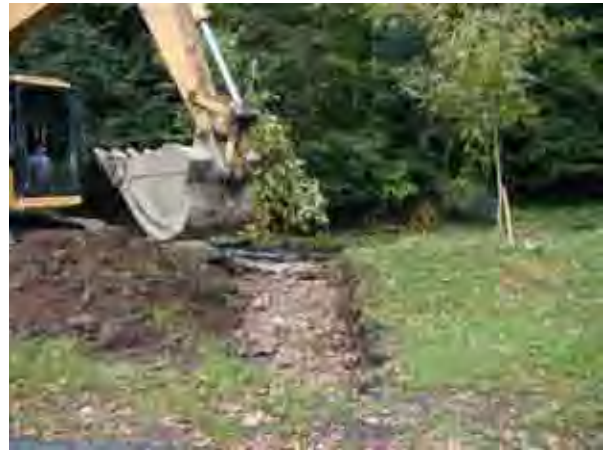
Photo 6. Swale expanded and filled with cobble; September 26, 2003.
