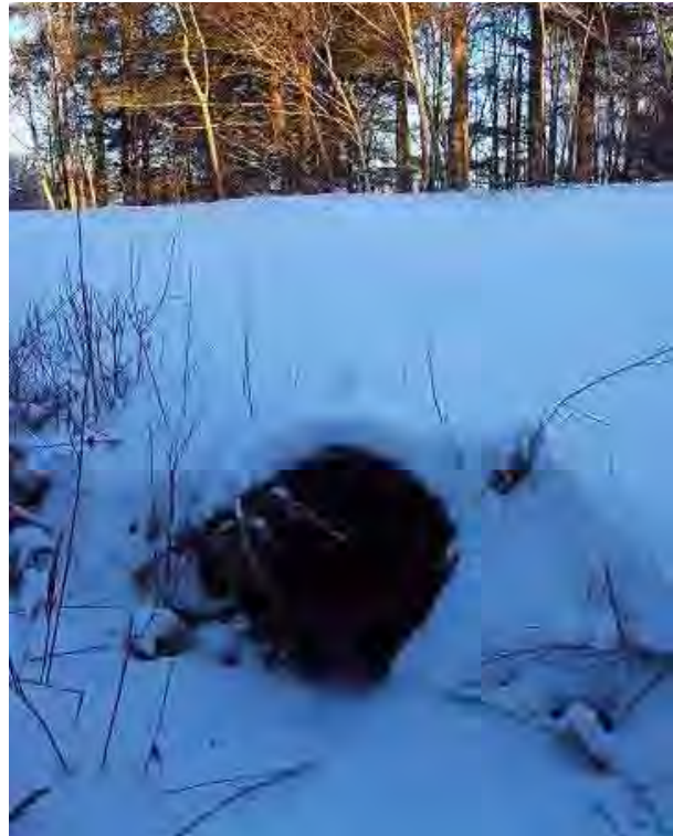
Photo 13. Tributary through culvert, Mutton Hill Rd.
