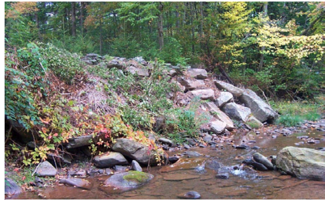
Photo 5. "New" dumped boulder rip-rap on right bank, just downstream from eroding bank section. Stream flow is from right to left.
