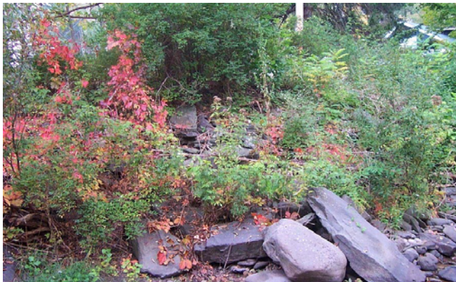
Photo 8. Mixture of dumped rock fill and laid up stone, with some vegetation colonizing the bank, just upstream from Rte. 28 bridge. Stream flow is from right to left.
