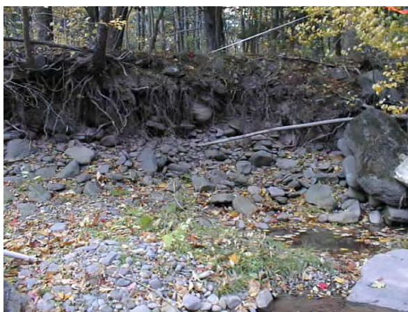
Photo 12. Eroding right bank, monitoring cross-section 2, at forested terrace, just upstream from hardened banks with boulders and concrete slabs. Stream flow is from right to left.
