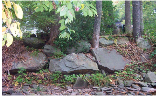
Photo 7. "Laid up" boulders along the right bank in the middle of MU18. Note trees with buried trunks. Stream flow is from right to left.
