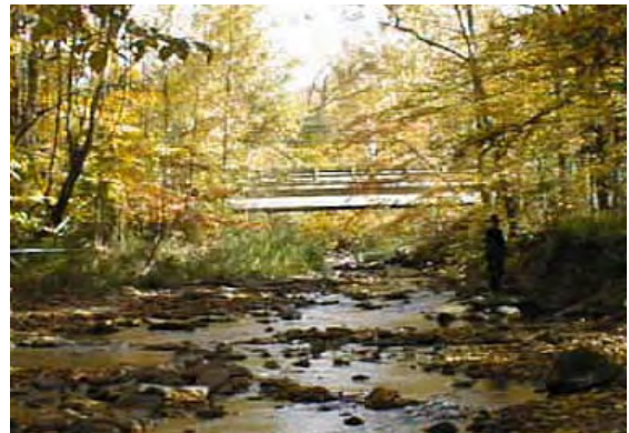
Photo 3. Looking upstream at bridge crossing NY State Route 28. MU18 ends just downstream from the bridge.
