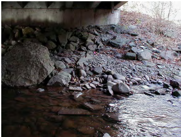
Photo 4. Right abutment of Rte. 28 bridge, showing gravel bar forming within the abutments, narrowing and deepening the active channel to improve sediment transport capacity, and reducing potential for further maintenance. Stream flow is from right to left.
