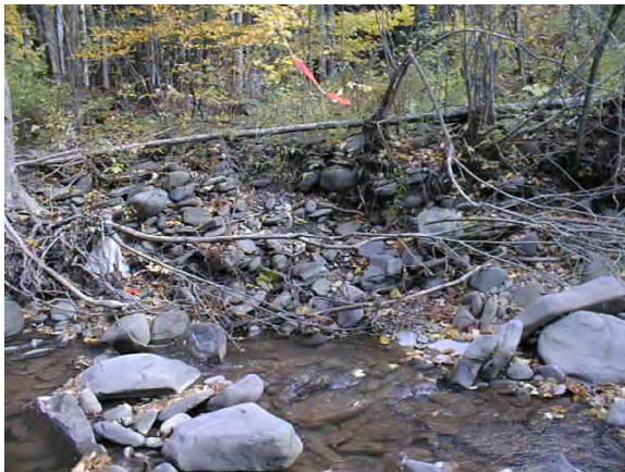
Photo 10. Pushed up material forming a berm along the left bank, just downstream from the berm shown in Photo 8, and opposite the eroding bank area documented in MU18. Stream flow is from left to right.
