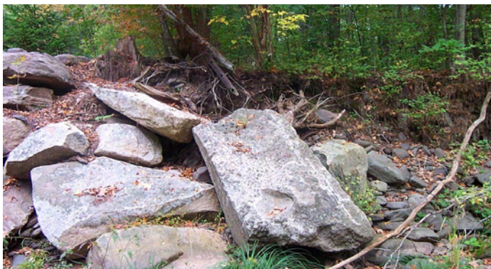
Photo 6. Upstream end of "new" boulder rip-rap section shown in Photo 5, with bank erosion just behind the end boulders, continuing upstream. Note trees eroding just behind, on the terrace. Stream is behind the viewer, flow is from right to left.
